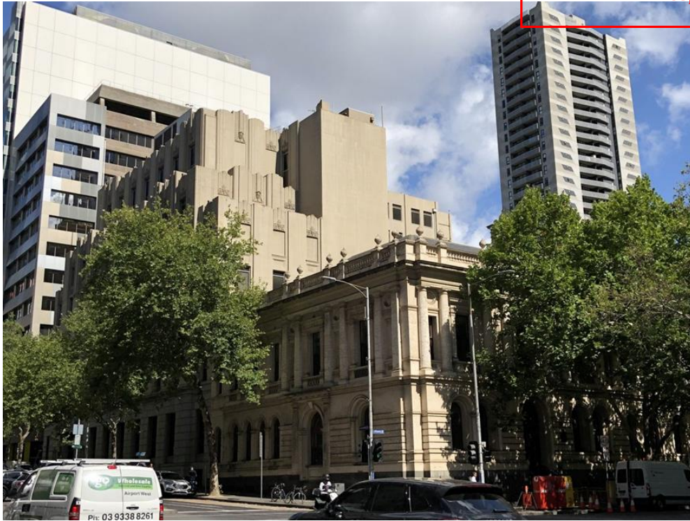
Figure 20 Oblique view west to the eastern façade of the subject building as viewed from the intersection of Lonsdale and Queen streets
