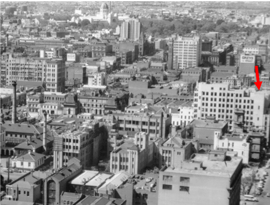
Figure 13 [Detail] View looking north-east, 1938: by this time the Taxation office (indicated) had been extended vertically by three levels and a caretaker's cottage had been added to the roof.
