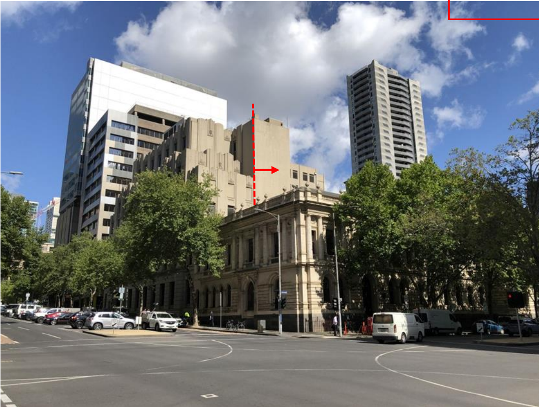
Figure 26 View of the subject site from the corner of Lonsdale and Queen Streets showing the eastern elevation, with the proposed extent of demolition indicated
