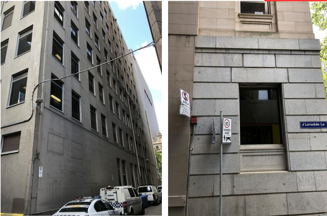
Figure 18 The western elevation as viewed from Lonsdale Lane (left) and detail of the return from the front façade (right)
