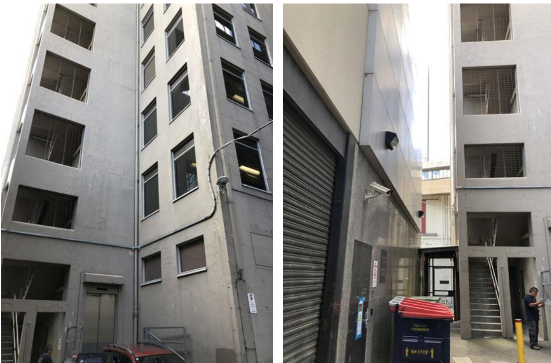
Figure 19 The external stairwell and north (rear) elevation of the building
