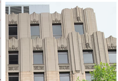
Existing heritage podium details
