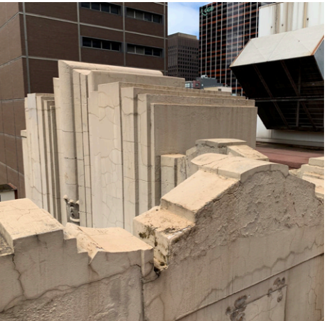
Existing parapet details
