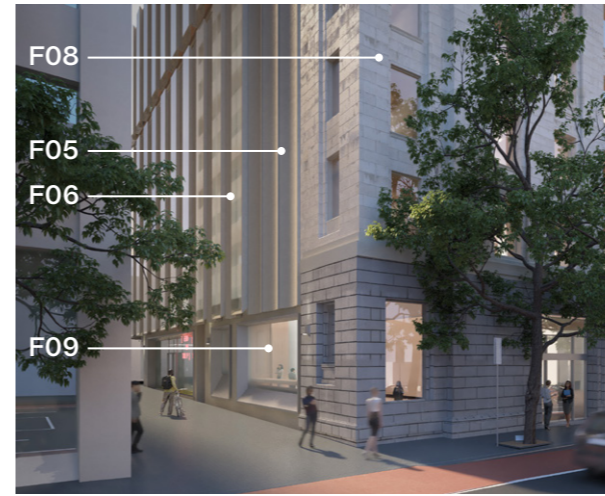
View to Lonsdale Lane
