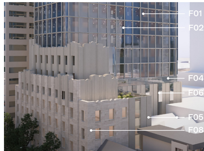
Elevated view of south-east podium corner
