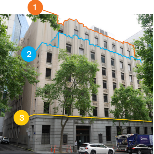
Existing heritage facade of 436 Lonsdale Street
