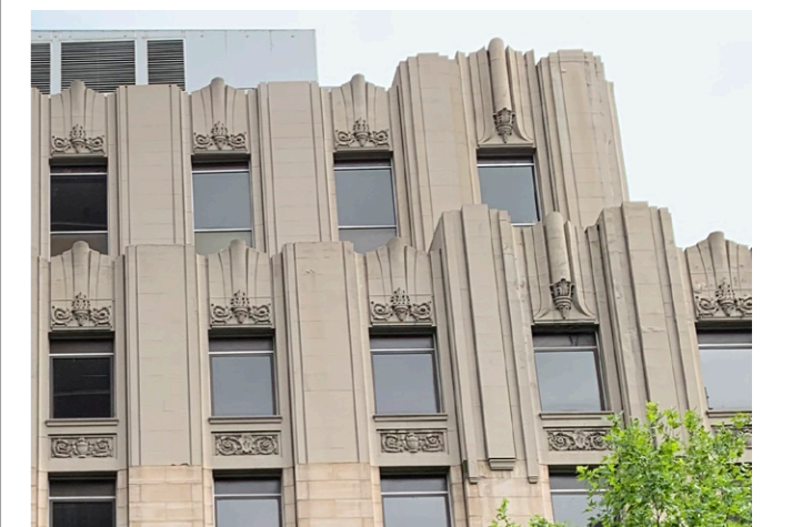
Existing heritage podium details
