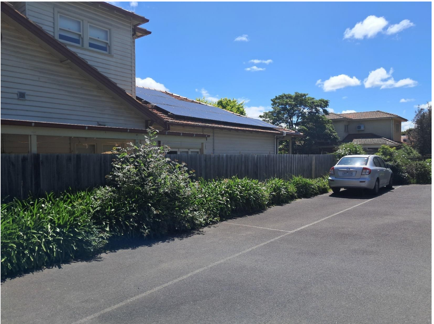
Figure 18: Existing solar panel facility adjacent to eastern boundary
