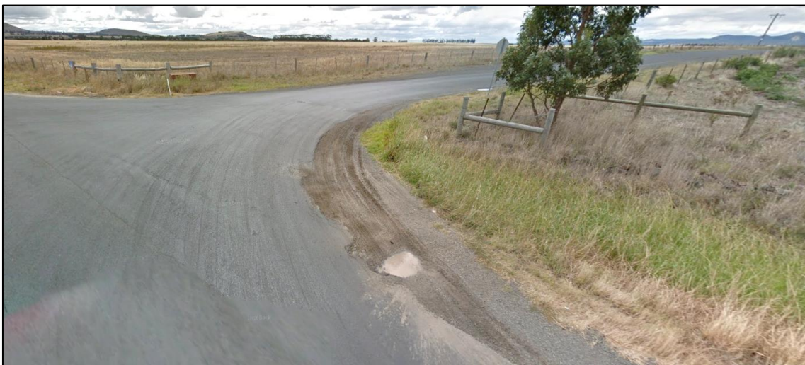
Figure 11: Geelong-Ballan Road Looking Northeast Towards Carrs Road Showing Damage at Edge of Seal
