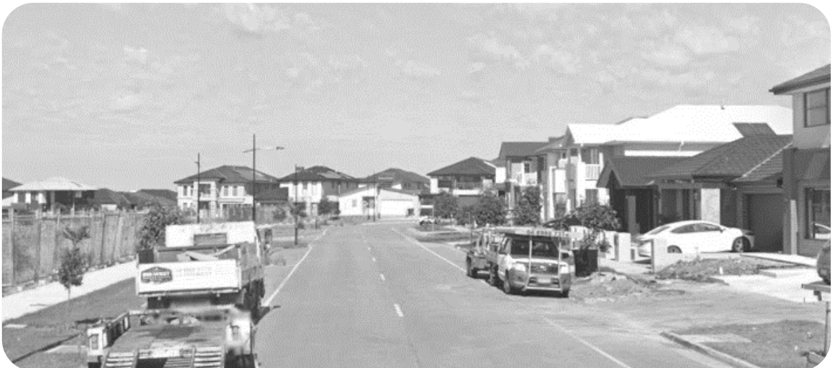
Figure 5 View of Carpathians Street facing south adjacent the subject site
