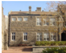
h00019 melbourne grammar school st kilda road melbourne cuming wing east she project 2004
