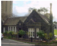
h00019 melbourne grammar school st kilda road melbourne lodge south elevation she project 2004
