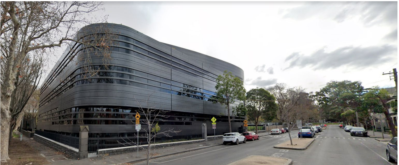
Picture 9 The Hanbury Science and Technology Centre viewed from the south-east.
