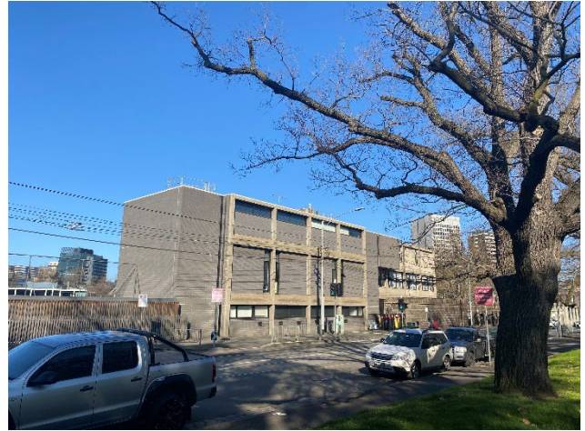
Picture 2 Existing Neill Building (viewed from the north-west)
