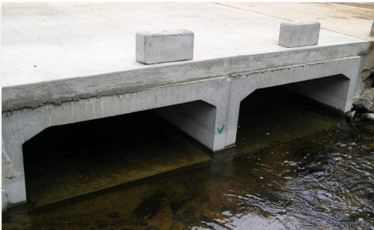
Figure 4: Multiple box culvert design
