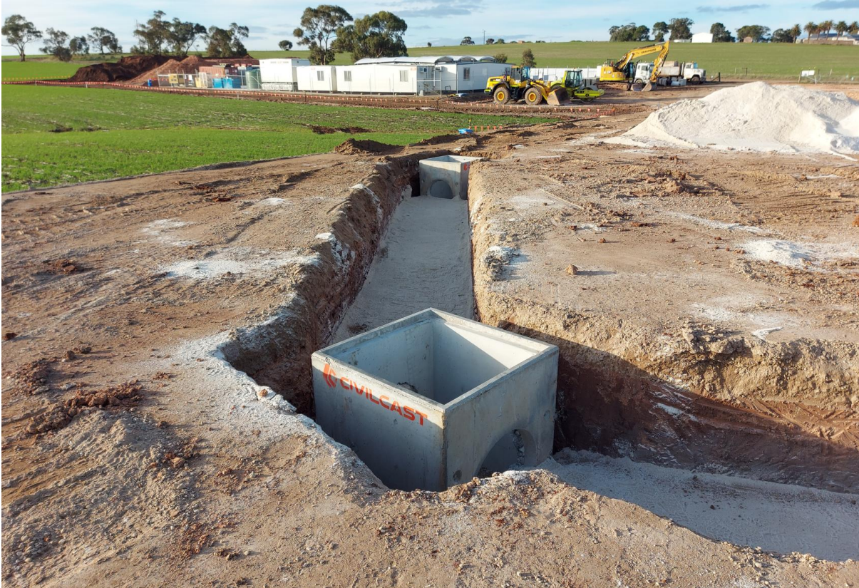
Figure 1: Drainage system under construction at Templers BESS in South Australia
