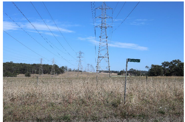
Figure 3-4 HV power line view from Parkins Road (looking east)
