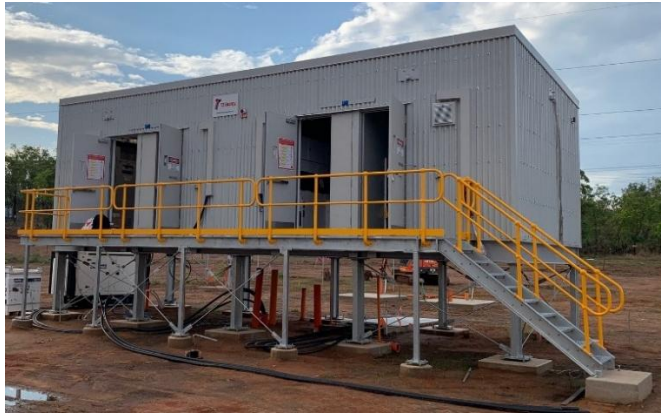
Figure 8 – Typical control building.
