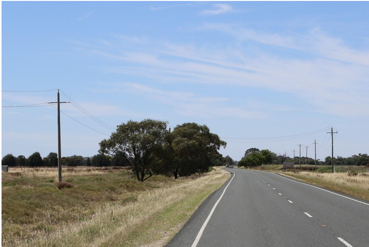
Figure 20 - Existing power lines adjacent to the Loddon Valley Highway at the western edge of the Project area.
