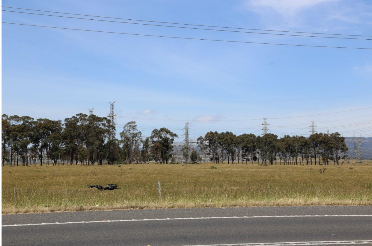
Figure 80 - Example of canopy vegetation providing visual integration of substation infrastructure.
