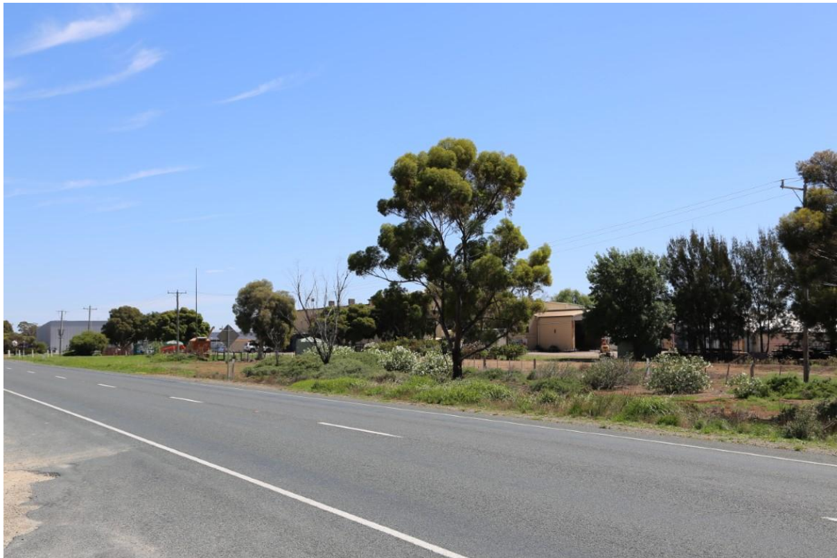
Figure 21 - View of the industrial area at the southern edge of Kerang.
