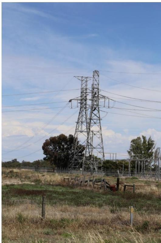
Figure 19 - HV Powerlines connecting to the Kerang Terminal Station traverse the landscape to the west of the Project area.
