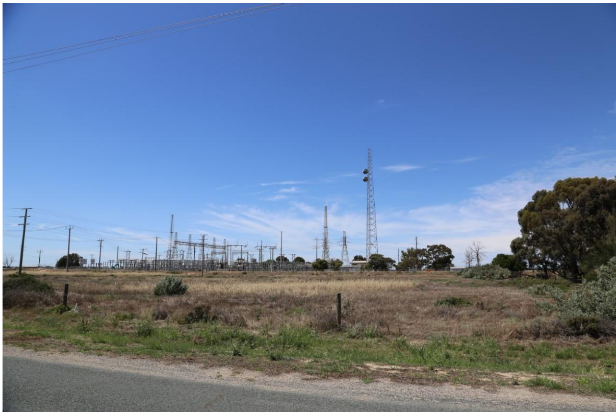
Figure 78 – V11 - View south southeast to the Project from Old Kerang Road (Photo VP11B).
