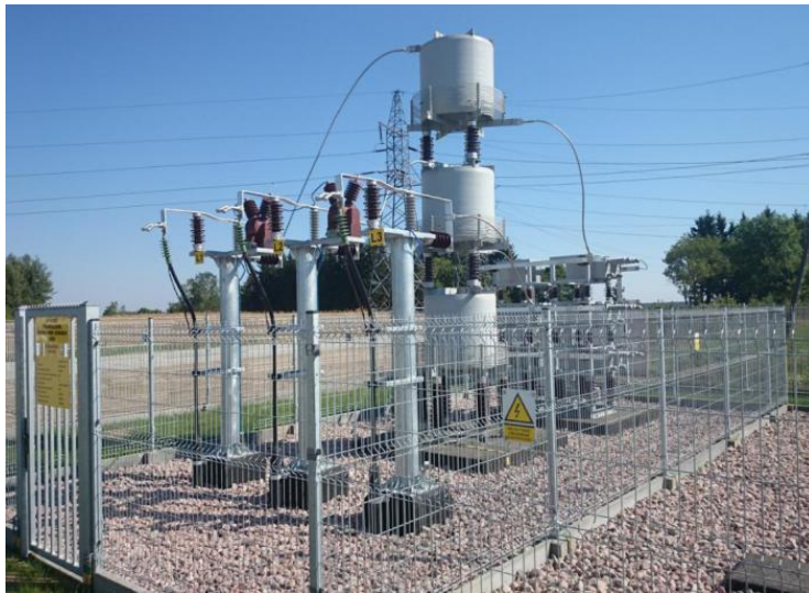
Figure 10 - Typical harmonic filter.
