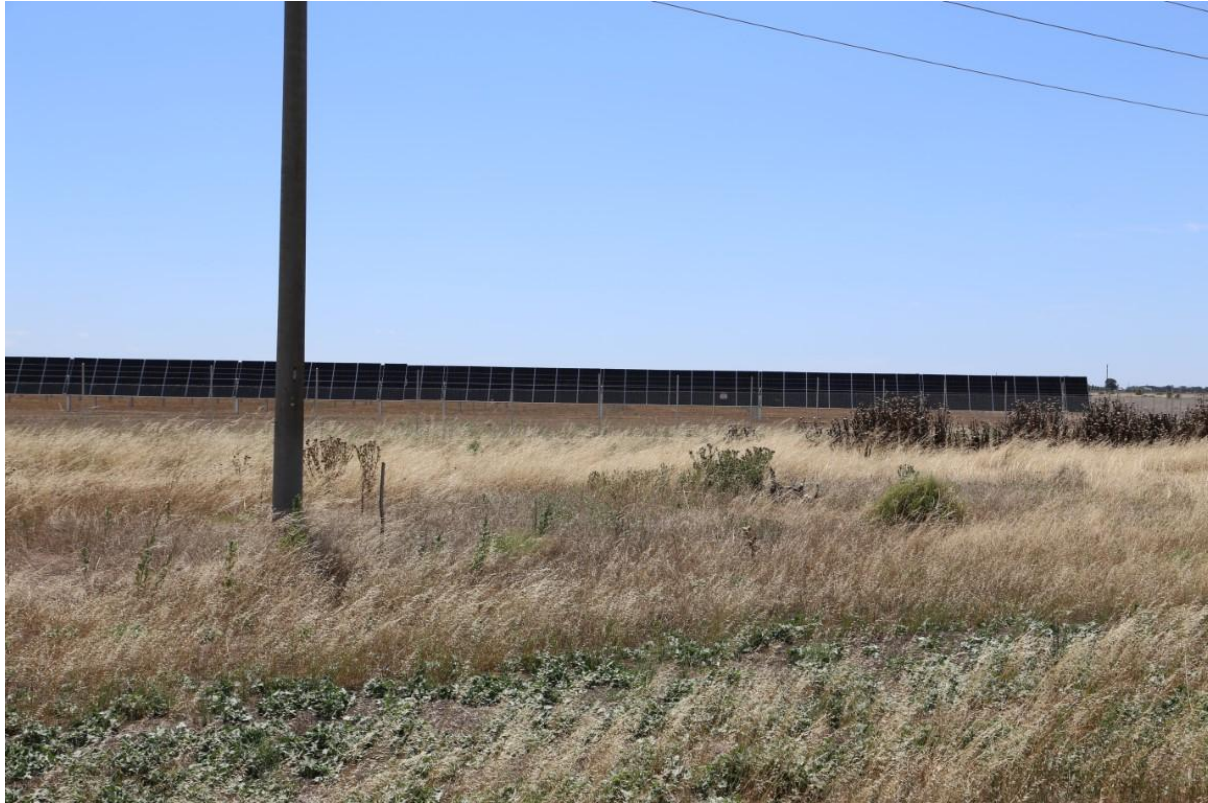
Figure 18 – The Kerang Solar Plant as viewed from the Loddon Valley Highway.
