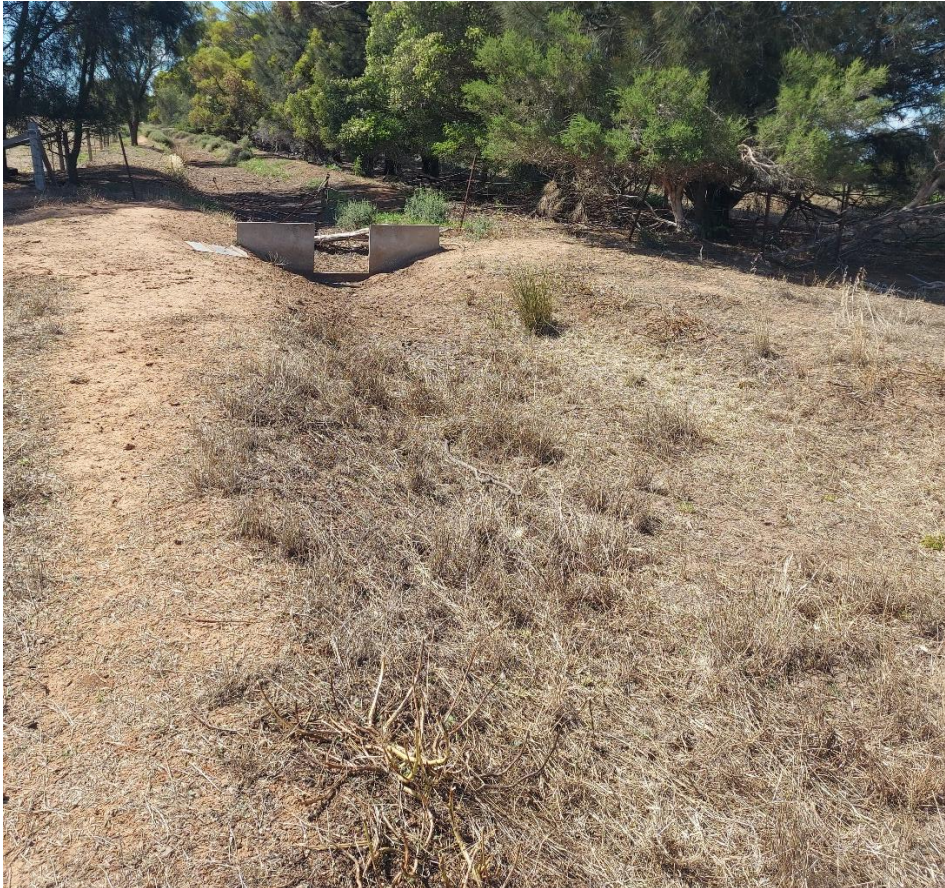
Figure 7. Image of Irrigation channel running south east to north west along the roadside boundary
