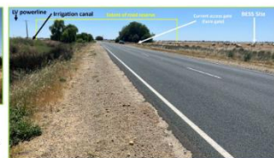
View looking north along Loddon Valley Highway towards the point where new junction will facilitate right turning into the BESS site.
