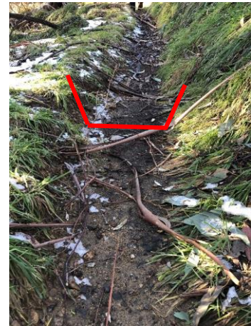
Plate 2 - Typical erosion of walking trail; noticeable 'valley' in trail.
