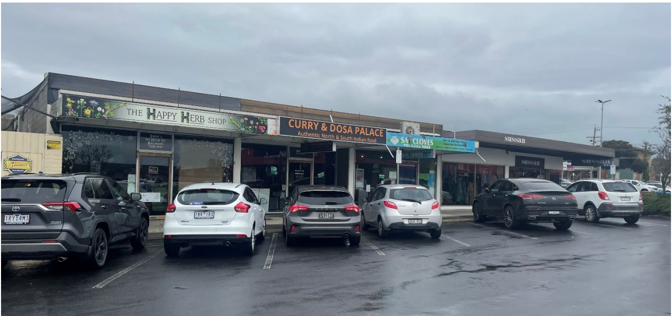
Figure 6. North-west facing shops at 164 High Street
