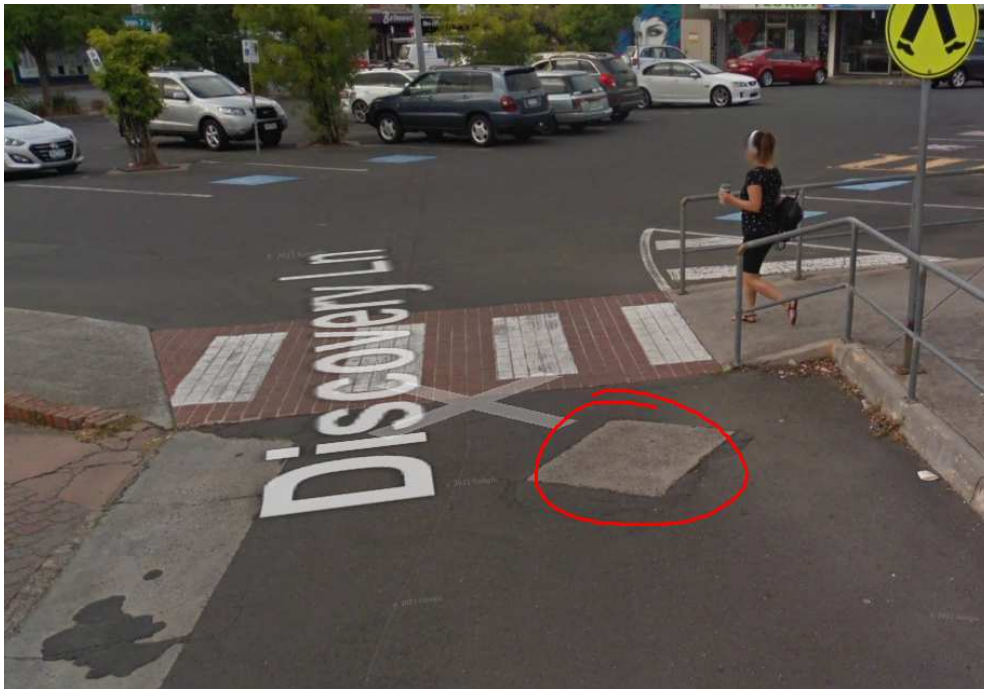
Figure 4 – Google Street View of Existing Pit in Discovery Lane
