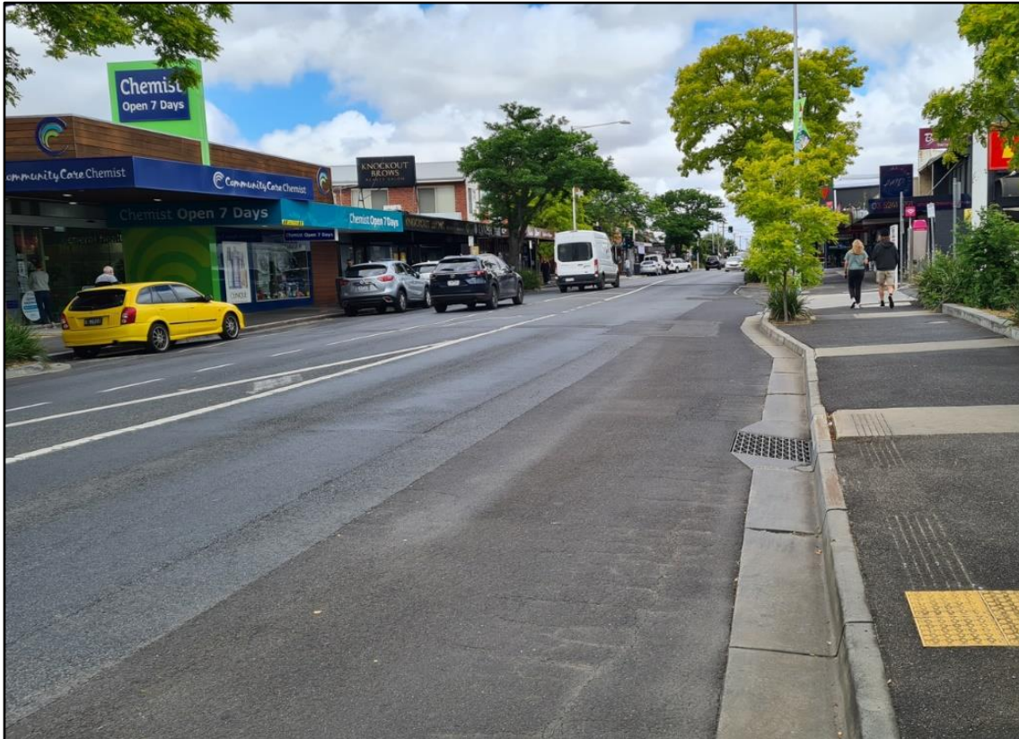
Figure 2.6: High Street, looking southwest
