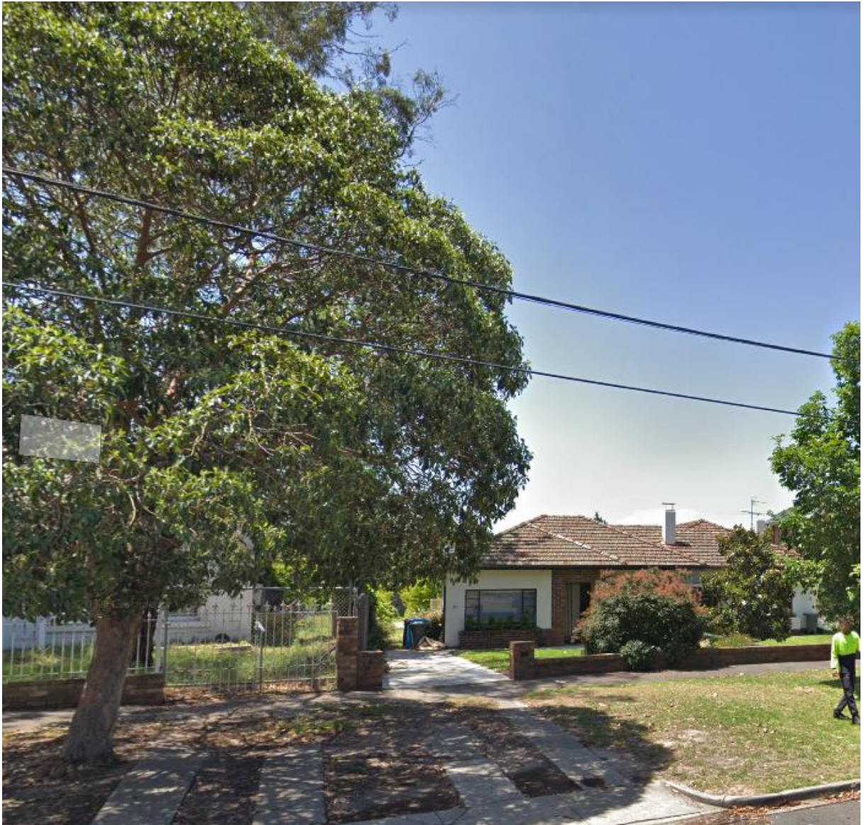
Figure 8 View of No. 8A and 8 Middle Crescent on the right viewed from Middle Crescent
