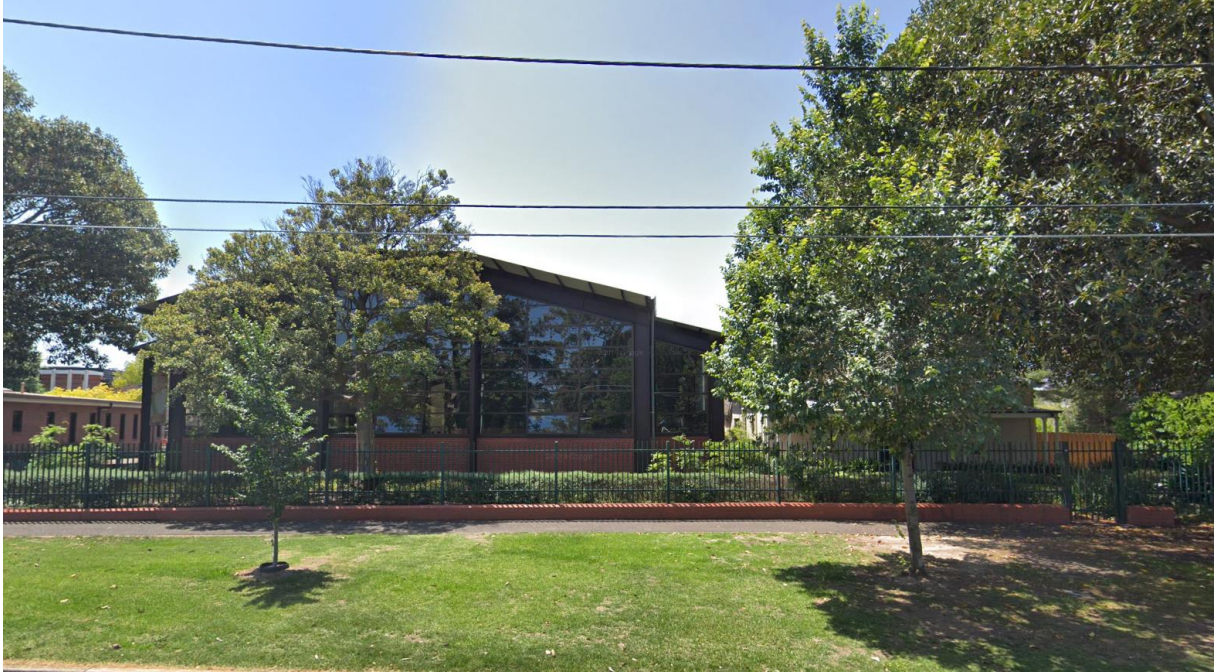
Figure 10 View of adjoining Physical Education Sports Centre and Seagrove House abutting site
