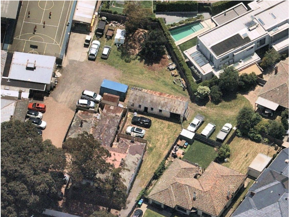
Figure 7 Aerial image of subject site bottom left, Firbank Grammar on the left, and No. 21 Anne Crescent at the top right
