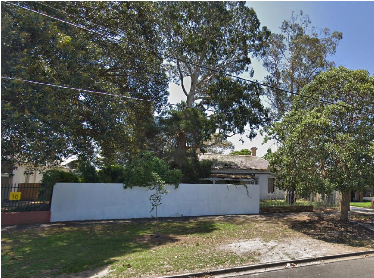
Figure 2 Subject site viewed from Middle Crescent
