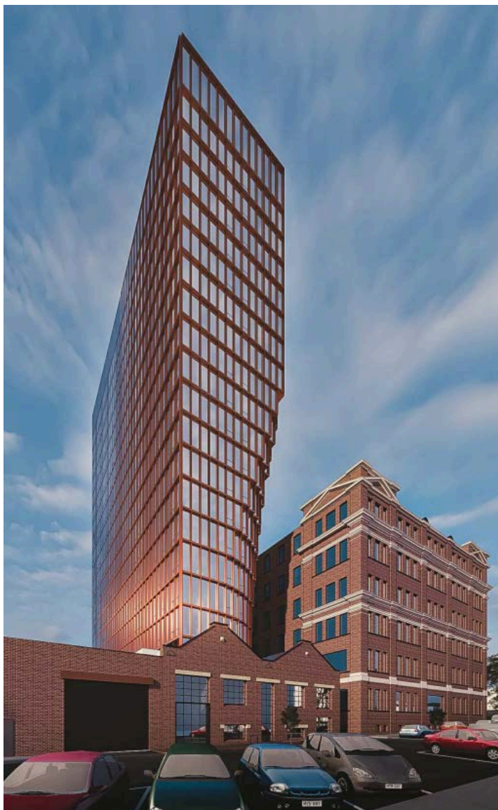
Figure 13: Extract of TP0.000 showing 3D render view of the new tower above the altered Jeffcott Street façade. Note the carved out lower level opening up views to the adjacent Sands & McDougall factory. Source: CHT Architects.
