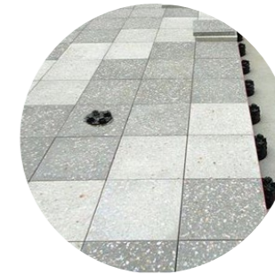
Precast pavers on a pedestal system (Level 19)
