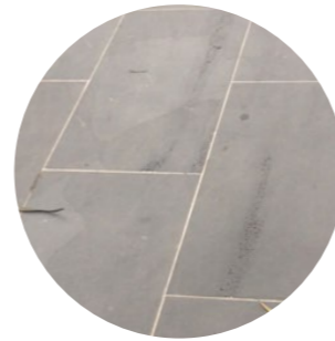
Large format bluestone pavers (Ground Floor)
