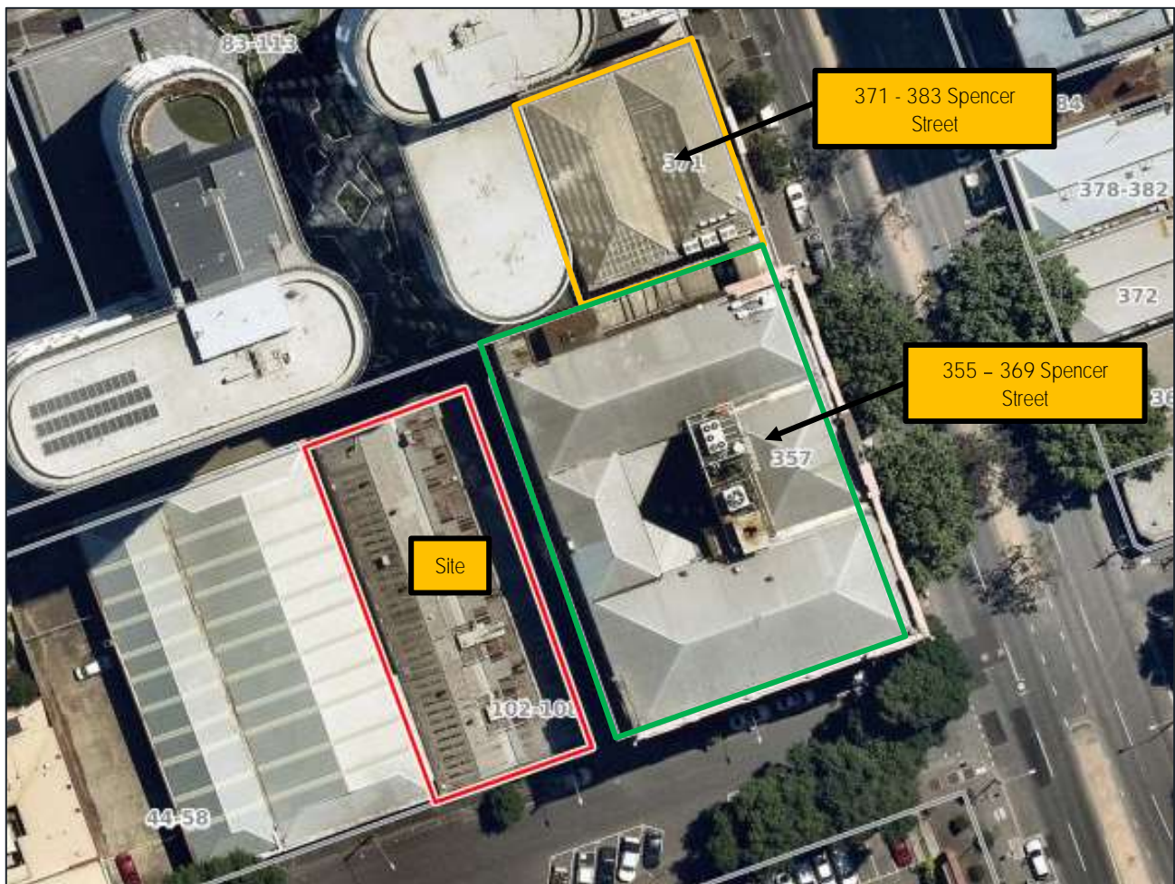
Figure 2 Aerial Photography of the Site, as well as the other properties affected by Planning Permit PA1800480. Source: www.onemap.com.au
