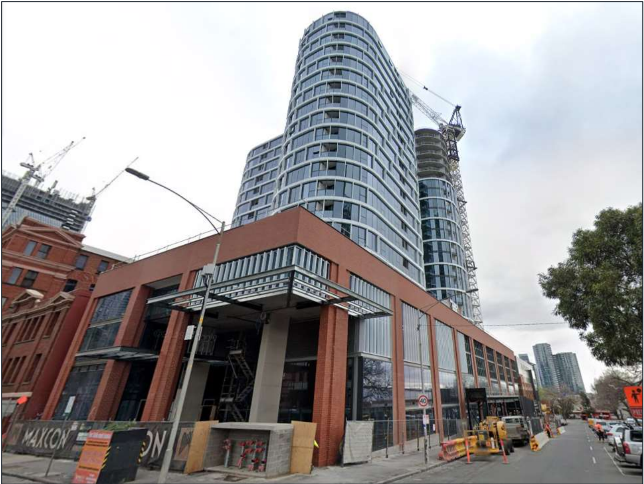
Image 4 – facing south west from the corner of Batman and Spencer Streets to the development at 83 – 133 Batman Street, Melbourne. Note that the development has now been completed – this image is from June 2019. Source: www.googlemaps.com.au
