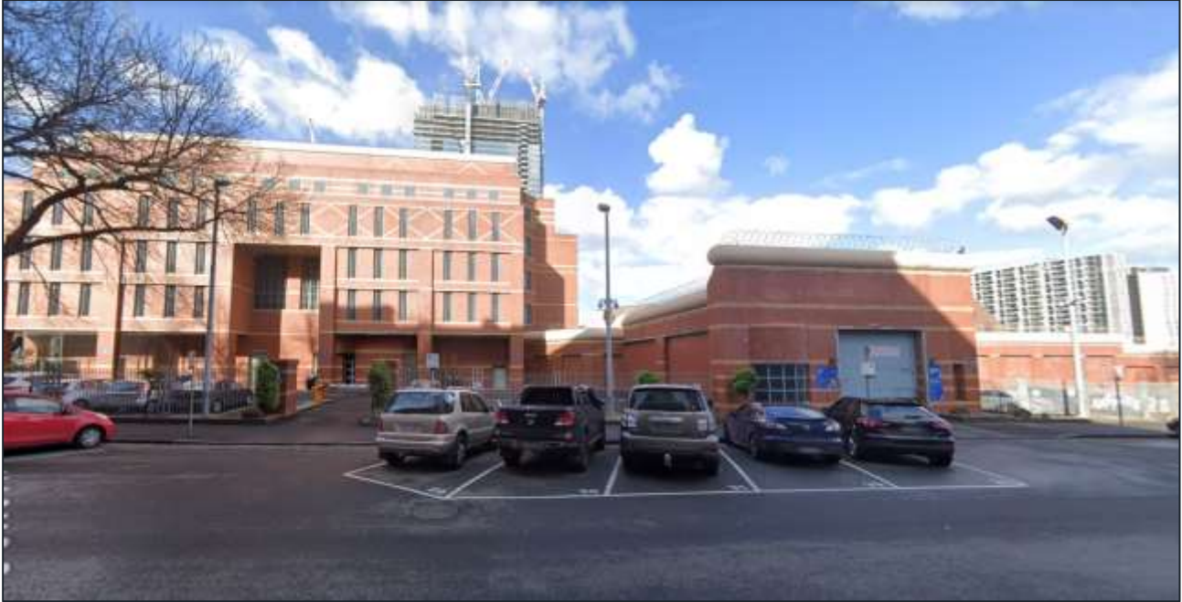
Image 6 – facing south from the Site to the Melbourne Assessment Prison. Source: www.googlemaps.com.au
