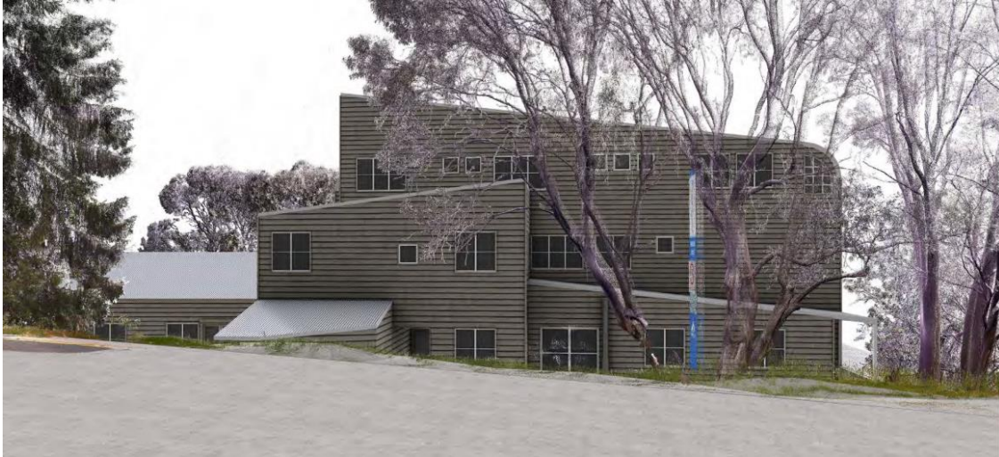
Figure 8 – Existing conditions – view from lower side of Arlberg Street – (Source: Application)
