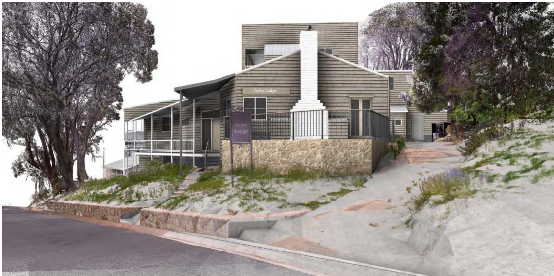
Figure 9 – Existing conditions – view from upper side of Slalom Street – (Source: Application)
