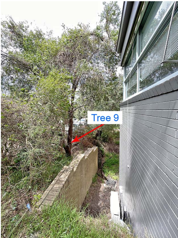
Image 4: Show the retaining wall south of Trees 8, 9 and 10 .
