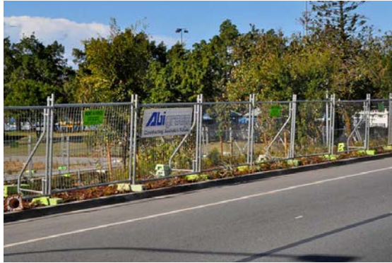
Figure 3: Tree protection fencing across a long section
