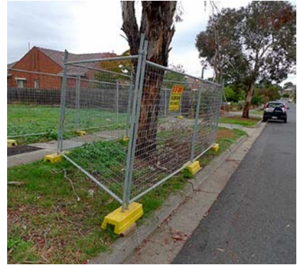
Figure 4: Tree protection fencing around a single tree in a nature strip setting.
