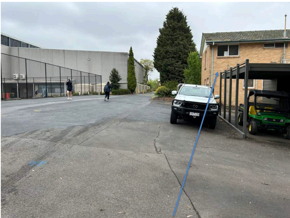
Photograph 8 - Existing archives building to be demolished
