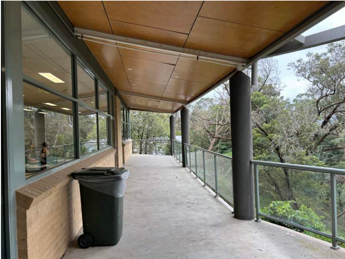
Photograph 3 - Existing senior school building - first floor verandah
