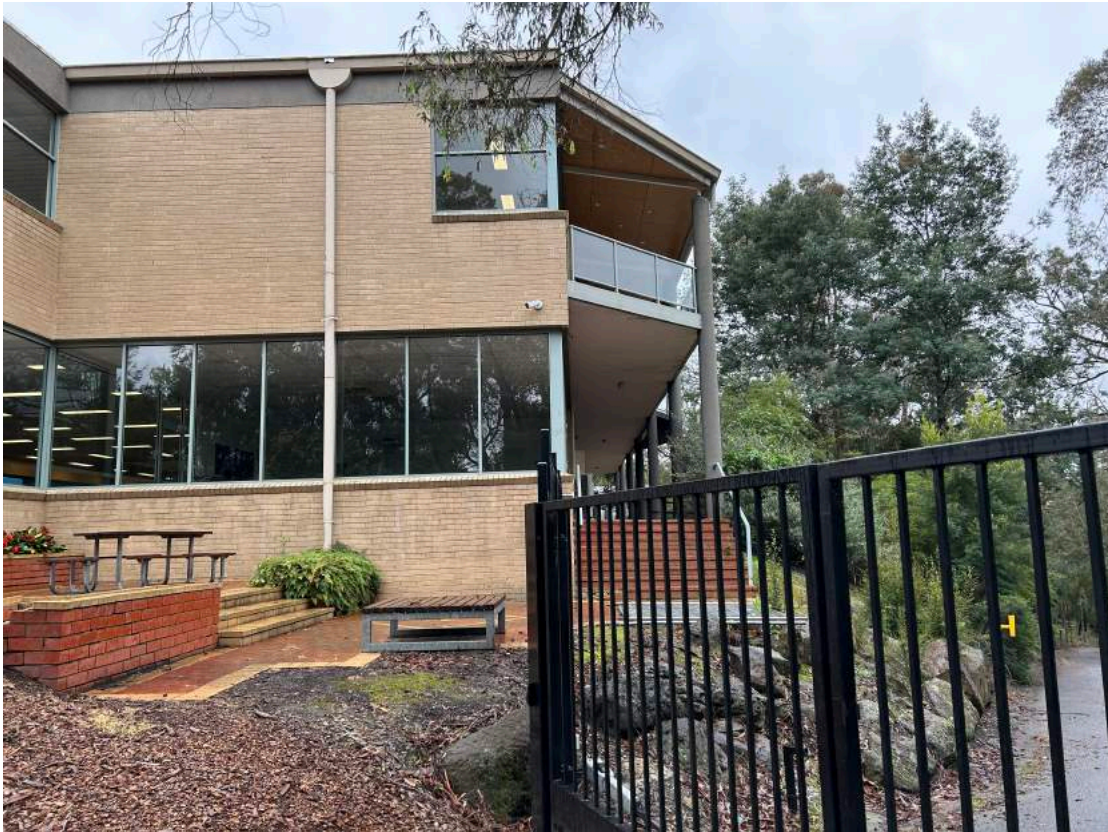
Photograph 1 - Existing senior school building
