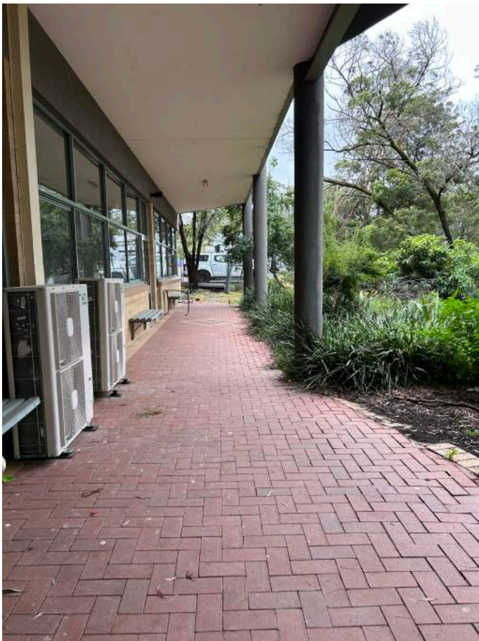
Photograph 2 - Existing senior school building - ground level verandah
