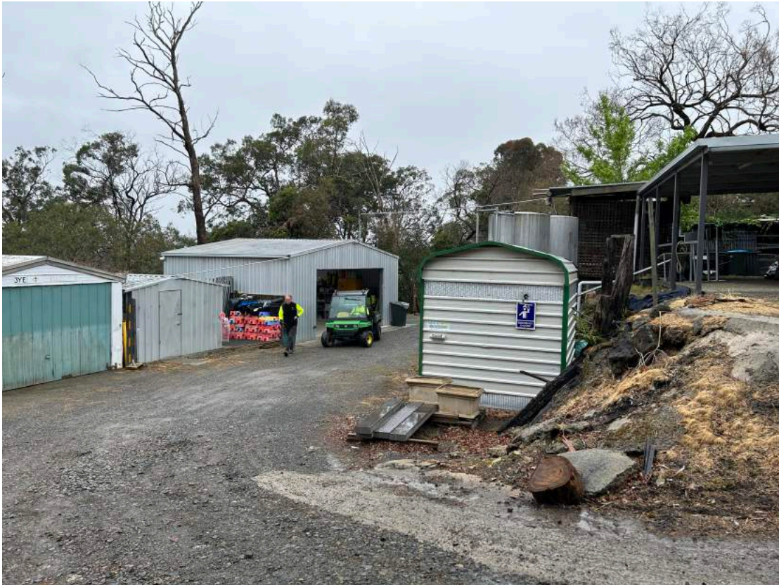
Photograph 13 – Existing facilities complex
