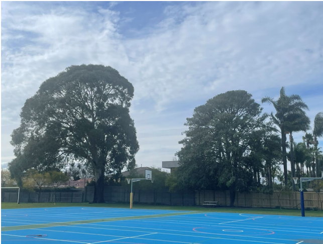
Figure 5 – Hardcourts within the proposed works area, looking east.
