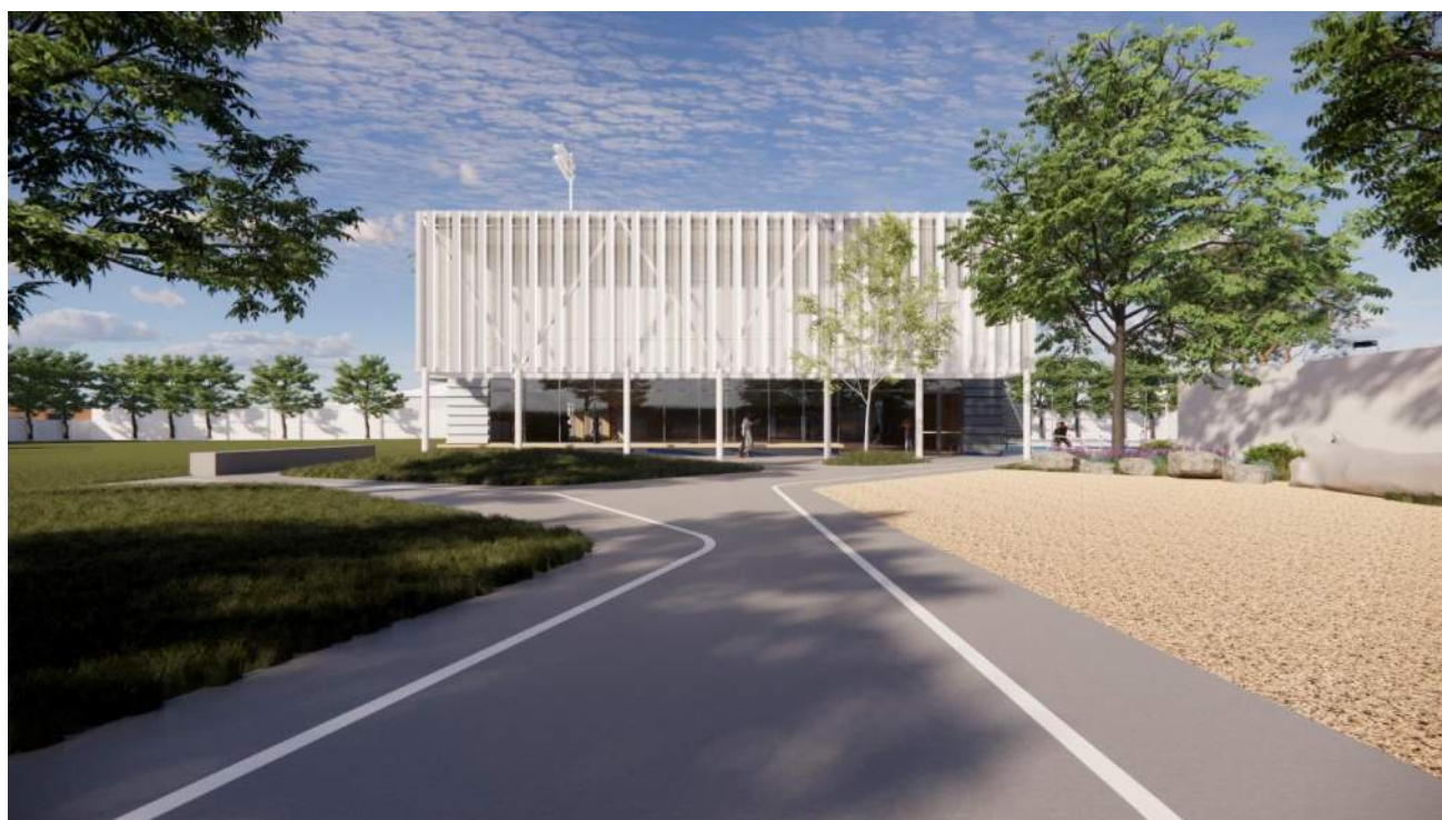
Figure 3 – Entry, West Elevation
