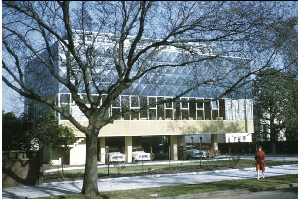
Figure 6 1958 image of the newly completed office building addition to the front of the original 'Blenheim' dwelling.
