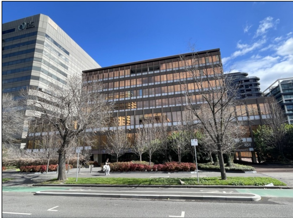
Figure 15 View of the St Kilda Road elevation of the VACC building.
