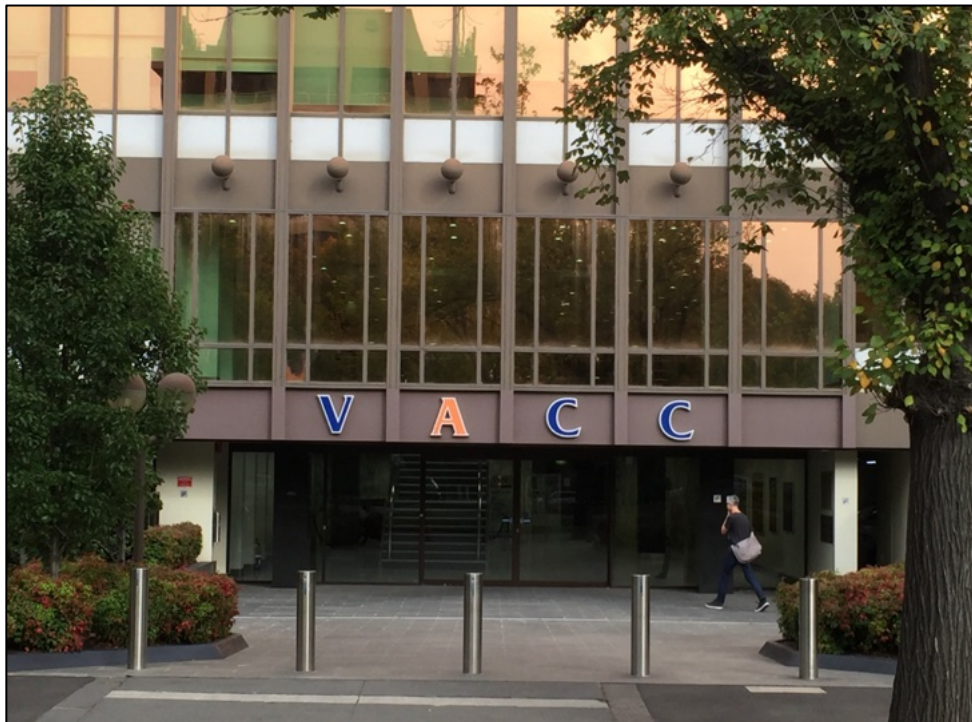
Figure 16 Detailed view of the entrance to the VACC building.
