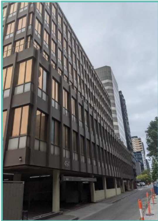
Picture 5 Rear of building with access to car parking shown
