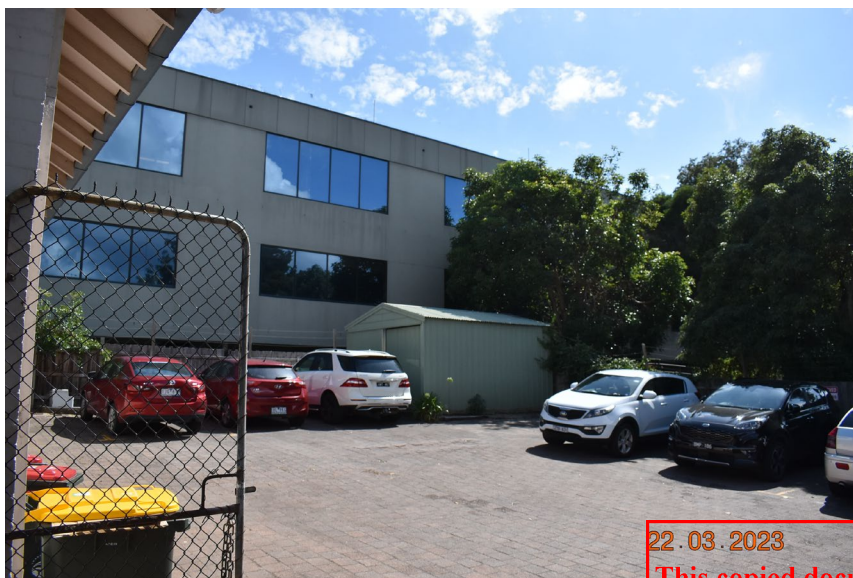
Figure 2: View of rear of 11 Beach Street, Frankston
