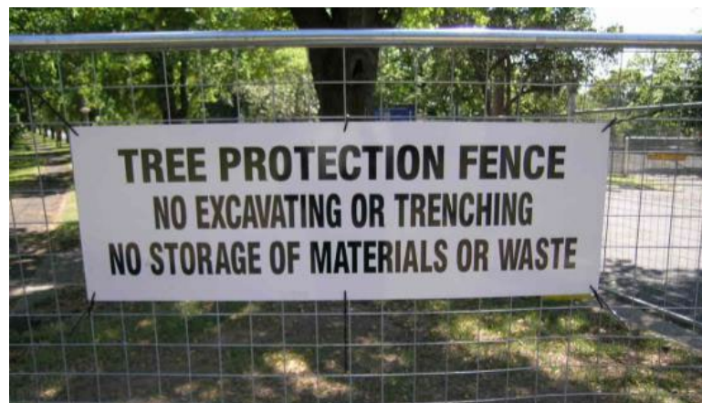
Figure 7: Example of a TPZ warning sign clearly displayed on TPZ fencing.
