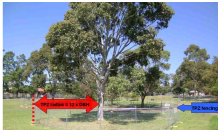
Figure 6: TPZ fencing is erected around retained trees prior to site works.
