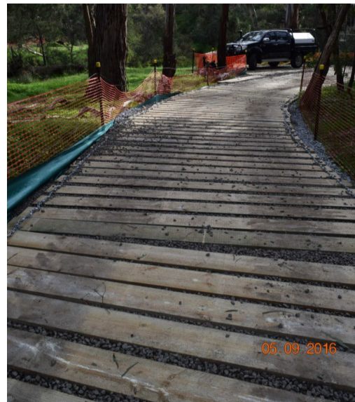
Figure 9: Rumble boards over crushed rock.
