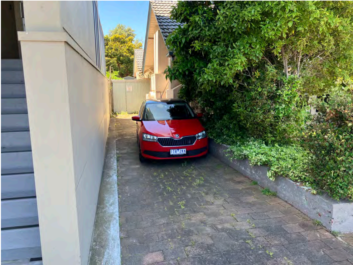
Figure 7. Western side of 11 Beach Street Frankston showing the significant ground disturbance.
