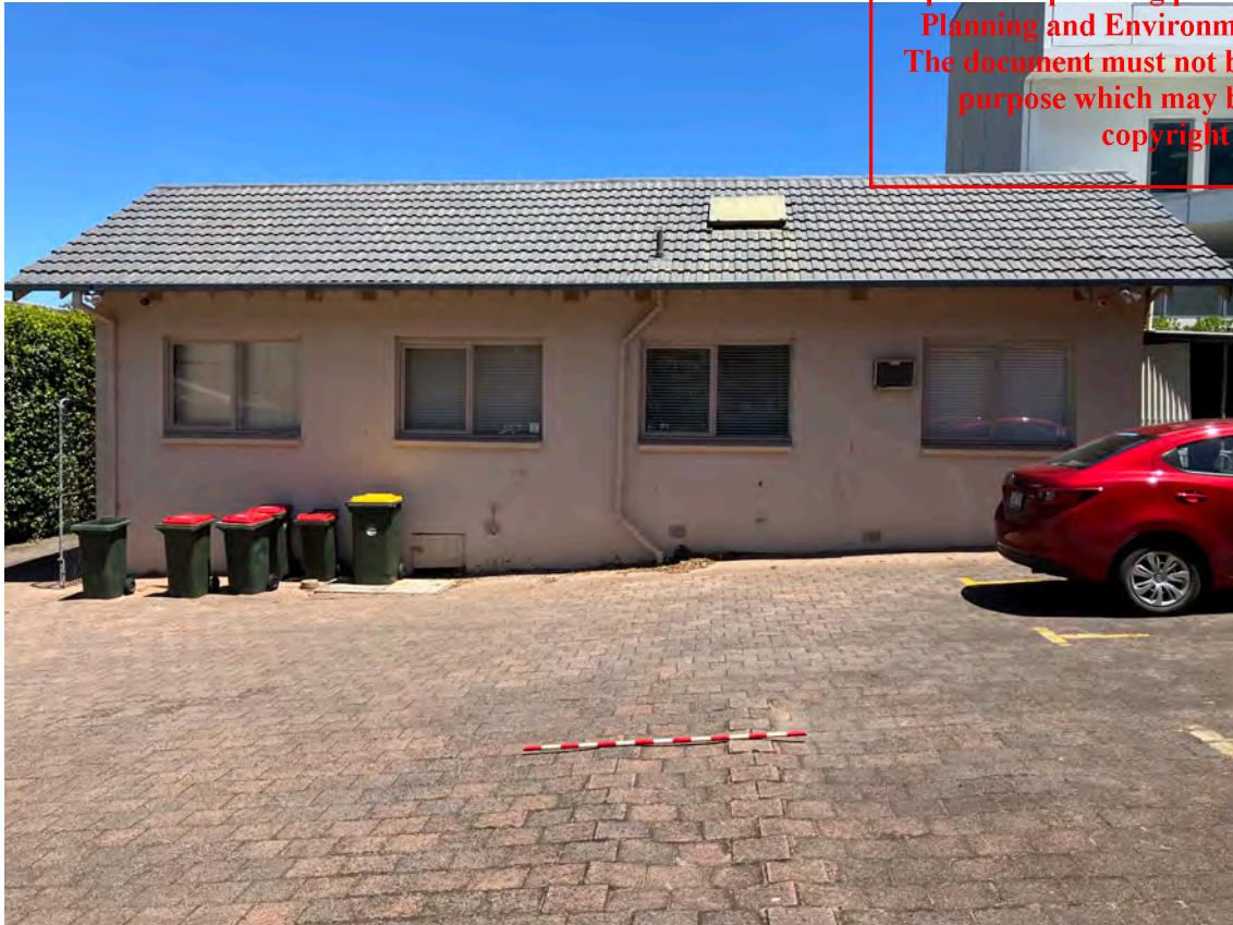
Figure 5. Rear of 11 Beach Street Frankston demonstrating the high levels of significant ground disturbance during concrete paving and dwelling construction.
