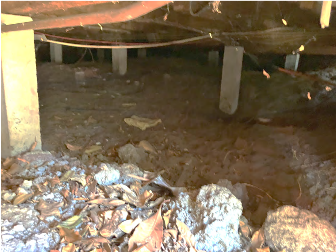
Figure 16. Underfloor cavity of 11 Beach Street Frankston.
