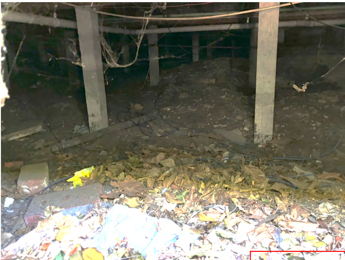
Figure 17. Underfloor cavity of 11 Beach Street Frankston.
