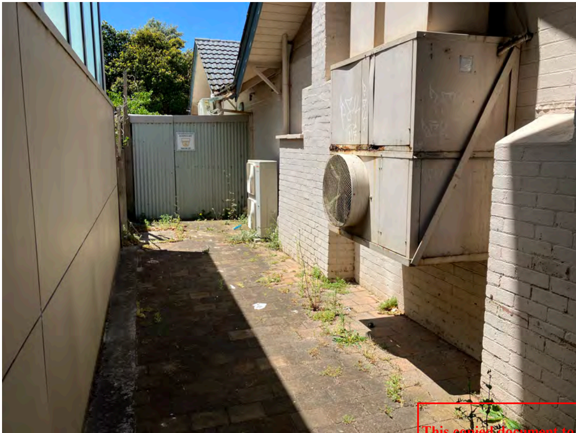
Figure 11. Western side of 11 Beach Street Frankston showing the significant ground disturbance.
