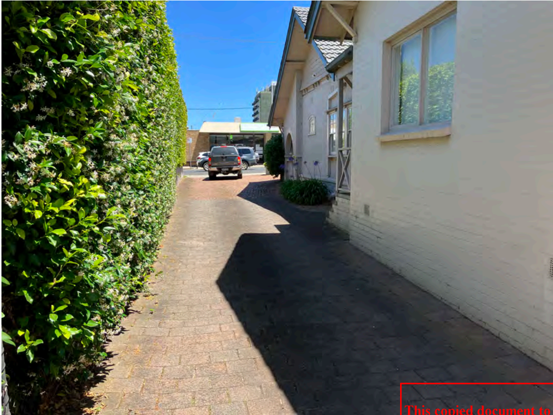
Figure 8. Eastern side of 11 Beach Street Frankston showing the significant ground disturbance.
