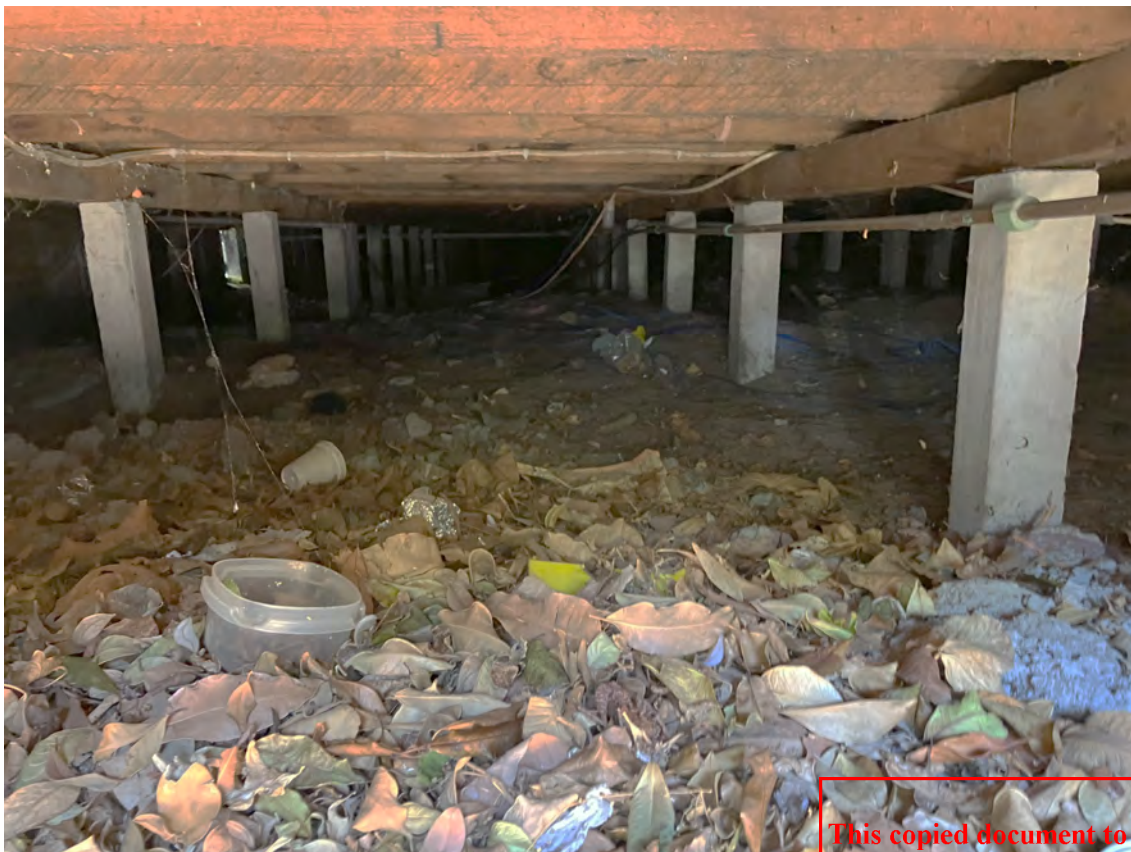
Figure 15. Underfloor cavity of 11 Beach Street Frankston.
