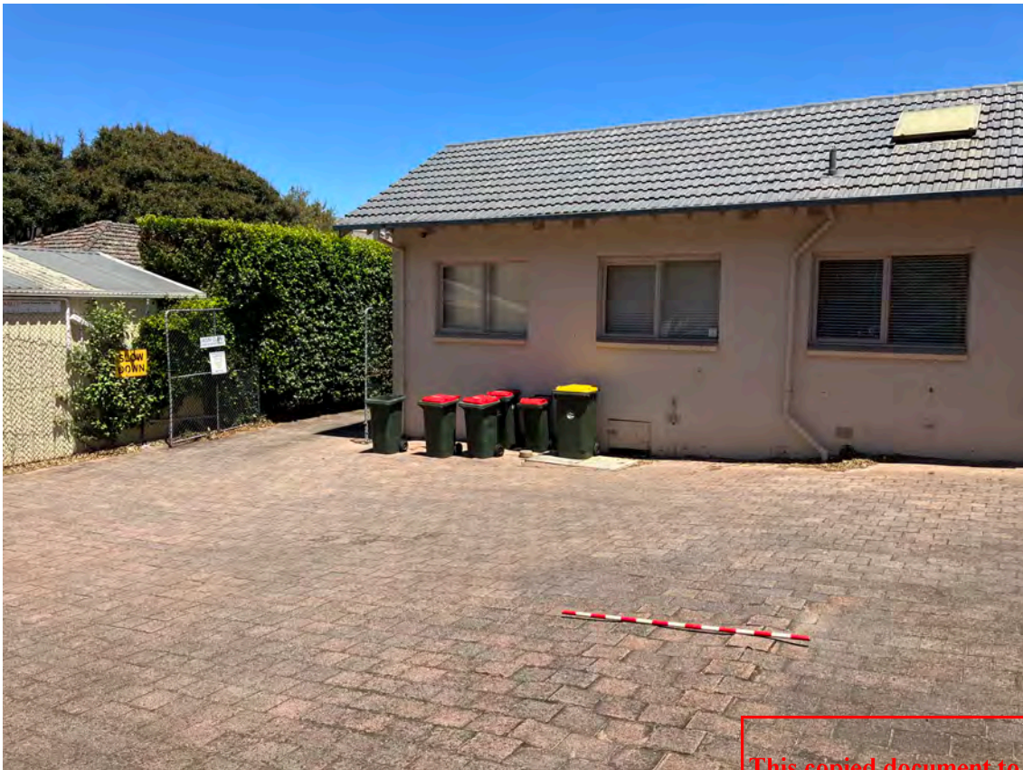
Figure 13. Rear of 11 Beach Street Frankston showing the significant ground disturbance. A large diameter sewer main has been trenching through this area.
