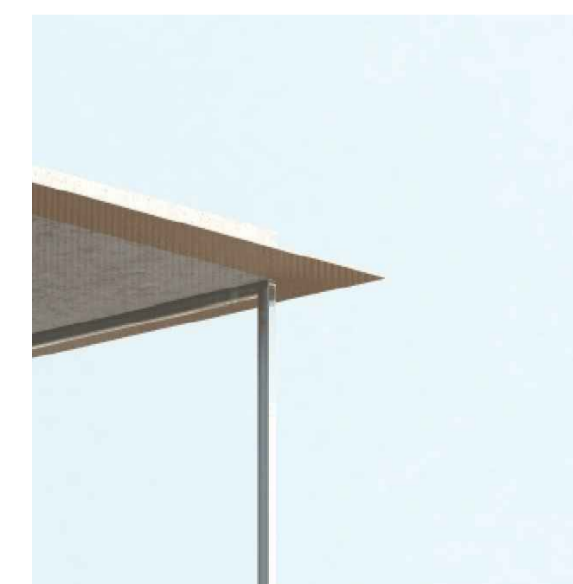
CODE: MT-01 DESCRIPTION: METAL AWNING MATERIAL: ALUMINIUM SHEET FINISH: POWDERCOATED COLOUR: NATURAL RED POWDERCOAT COLOUR
