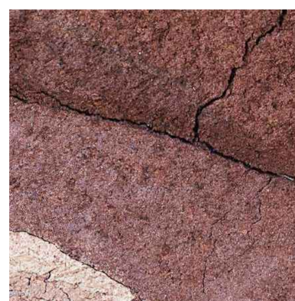
CODE: C-06 DESCRIPTION: ARCHITECTURAL CONCRETE MATERIAL: INSITU CONCRETE COLUMNS & SLABS FINISH: OFF-FORM FINISH CLASS 2 COLOUR: TERRACOTTA / NATURAL RED OXIDE COLOUR (INTEGRAL OXIDE COLOUR)
