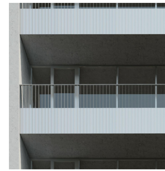
CODE: BAL-01 DESCRIPTION: BALUSTRADE MATERIAL: METAL BALUSTRADE NOM. 50x10 VERTICALS & TOP RAIL, SOLID INFILL PANEL COVERING SLAB EDGE AND EXTENDING TO 800H ABOVE FLOOR LEVEL FINISH: GALVANISED COLOUR: RAW GALVANISED
