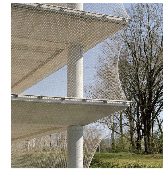
CODE: ME-01 DESCRIPTION: BIRD MESH MATERIAL: BIRD-PROOF STAINLESS STEEL WIRE TENSION MESH TO WIND VENTING LEVEL FINISH: STAINLESS STEEL COLOUR: NATURAL STAINLESS STEEL
