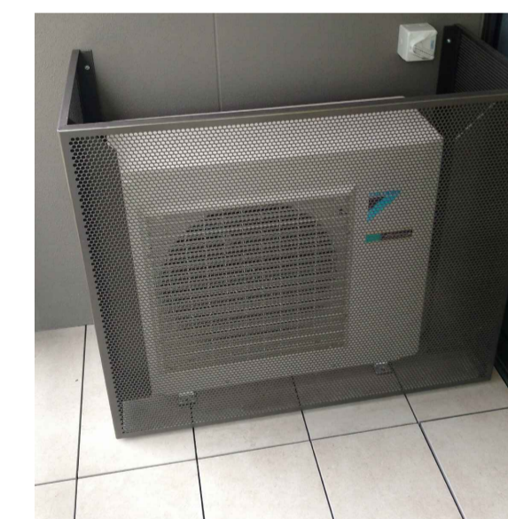
CODE: SCR-03 DESCRIPTION: A/C UNIT SCREEN MATERIAL: PERFORATED ALUMINIUM SCREEN FINISH: POWDERCOATED ALUMINIUM COLOUR: GULL GREY POWDERCOAT
