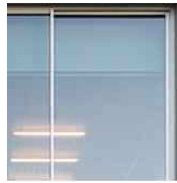
CODE: GLZ-01 DESCRIPTION: FACADE GLAZING MATERIAL: DOUBLE GLAZED WINDOWS IN POWDERCOATED ALUMINIUM FRAME (APARTMENTS) FINISH: LOW-E NEUTRAL GLASS / POWDERCOATED ALUMINIUM COLOUR: NEUTRAL GLASS COLOUR / GULL GREY POWDERCOAT
