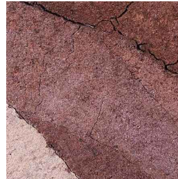
CODE: CFC-02 DESCRIPTION: EXTERNAL CLADDING MATERIAL: COMPRESSED FIBRE CEMENT CLADDING FINISH: RAW / NATURAL FINISH COLOUR: FULL-DEPTH THROUGH COLOUR IN NATURAL RED / TERRACOTTA TO MATCH C-03 COLOUR
