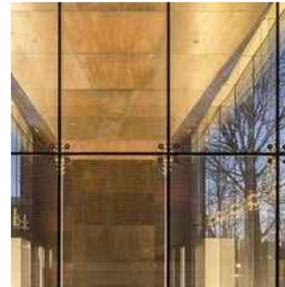
CODE: GLZ-02 DESCRIPTION: FACADE GLAZING MATERIAL: DOUBLE GLAZED WINDOWS IN POWDERCOATED ALUMINIUM FRAME (GROUND FLOOR) FINISH: LOW-E NEUTRAL GLASS / POWDERCOATED ALUMINIUM COLOUR: NEUTRAL GLASS COLOUR / TERRACOTTA COLOUR POWDERCOAT FRAME
