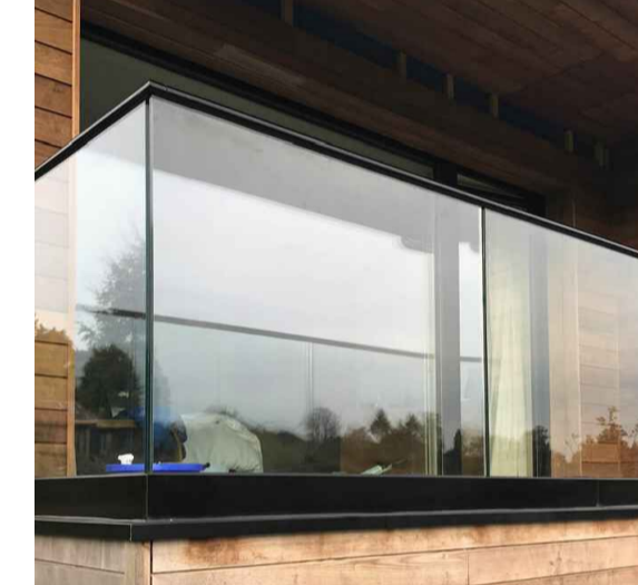
CODE: BAL-03 DESCRIPTION: BALUSTRADE MATERIAL: STRUCTURALLY GLAZED GLASS BALUSTRADE WITH ALUMINIUM POST & FRAME FINISH: CLEAR GLASS & POWDERCOATED ALUMINIUM COLOUR: SURFMIST POWDERCOAT COLOUR
