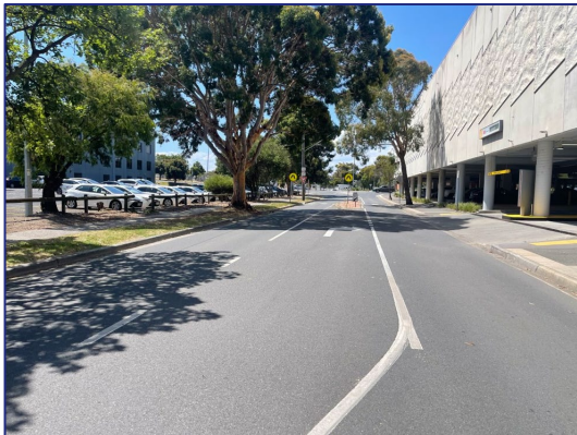
Figure 7: Evelyn Street – View North
