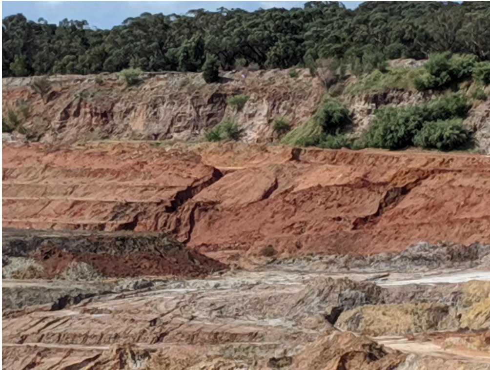
Figure 13 Example of Erosion of Exposed Sand Batters at Nearby Quarry
