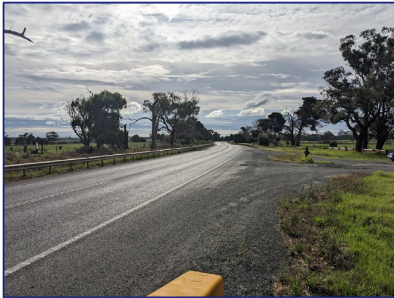
Figure 3: South Gippsland Highway - View North
