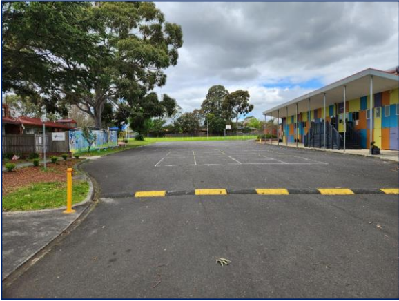
Figure 8: Informal Car Parking Area
