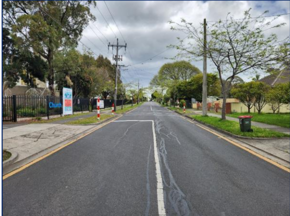
Figure 4: Stevens Road - view south
