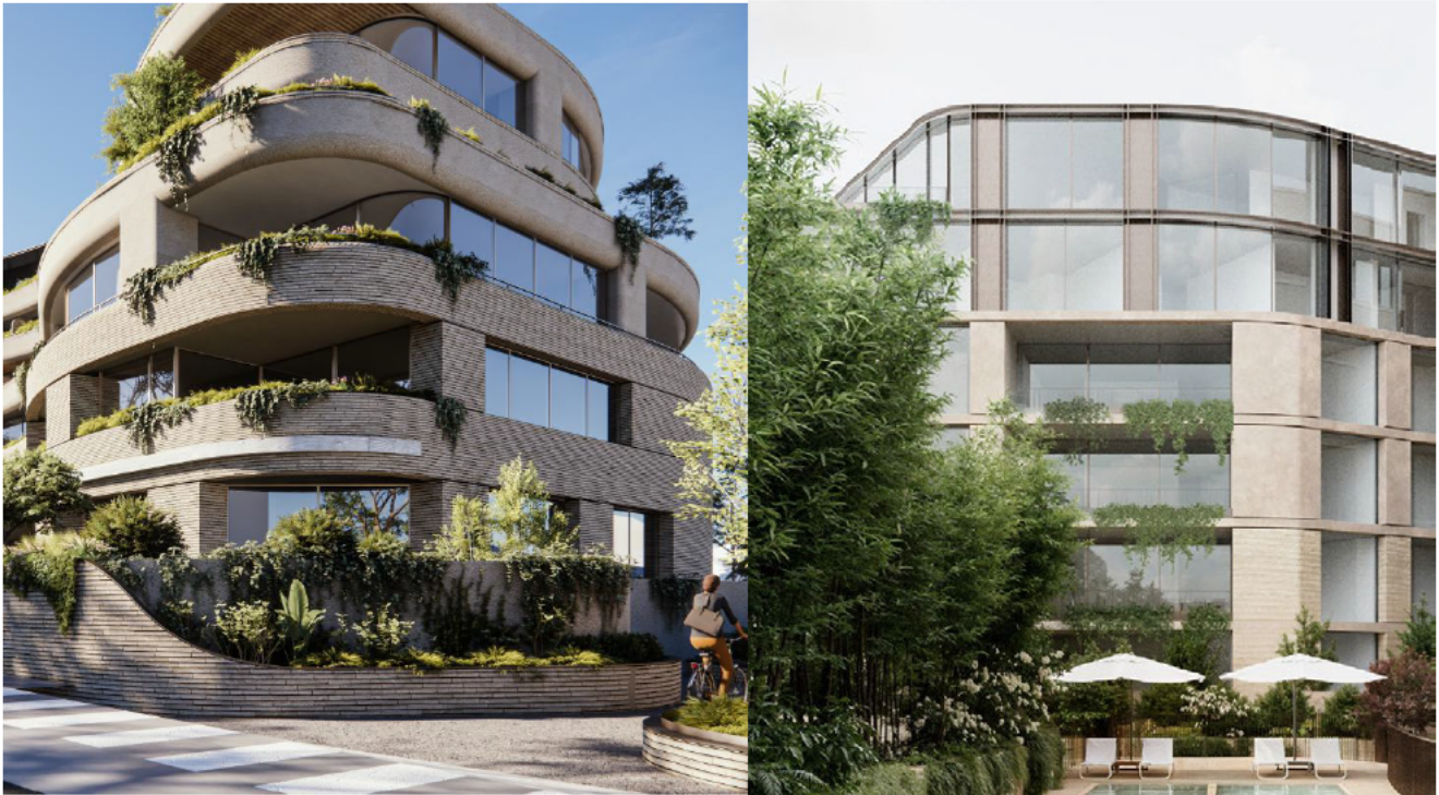
Figure 33 – 3D renders demonstrating proposed material palette, including brick and textured render material (left) and bronze metal cladding to upper floors (right)
