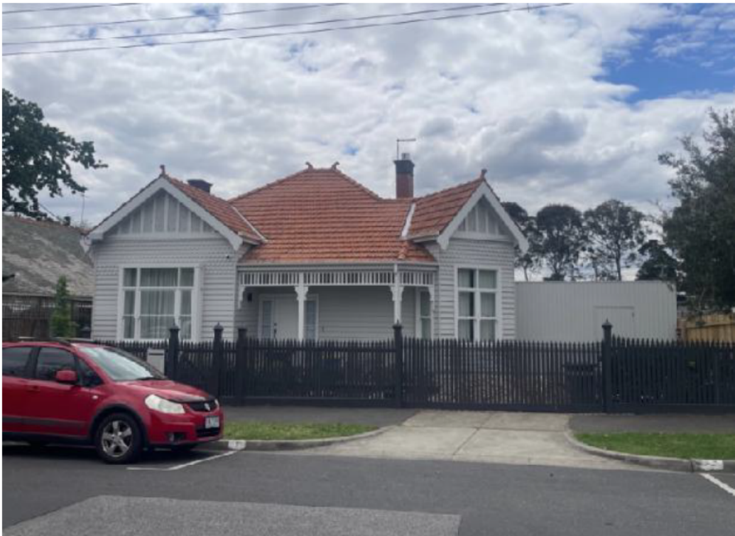
Figure 22 – The contributory dwelling at 11 Hawthorn Grove to the west of the site, including recent building addition abutting the shared boundary.
