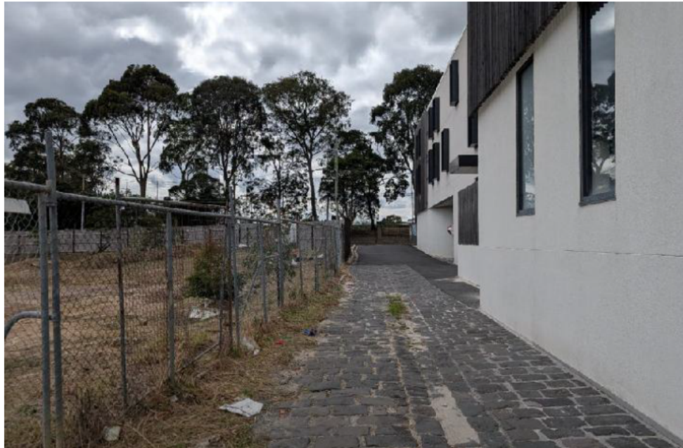
Figure 20 – Interface of childcare centre with the site’s eastern boundary (cobblestone laneway is the E1 easement portion of the laneway which is within the site’s title boundaries.
