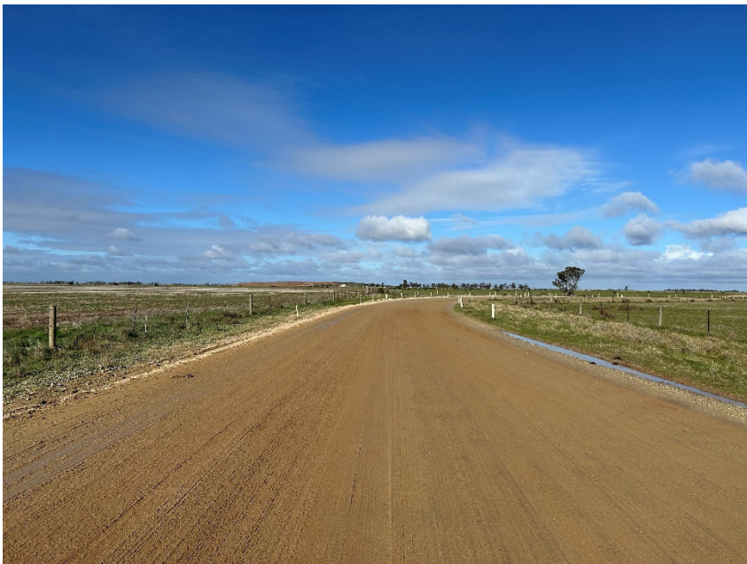
Figure 5: Davis Road, view to south. Subject land to left of photo.
