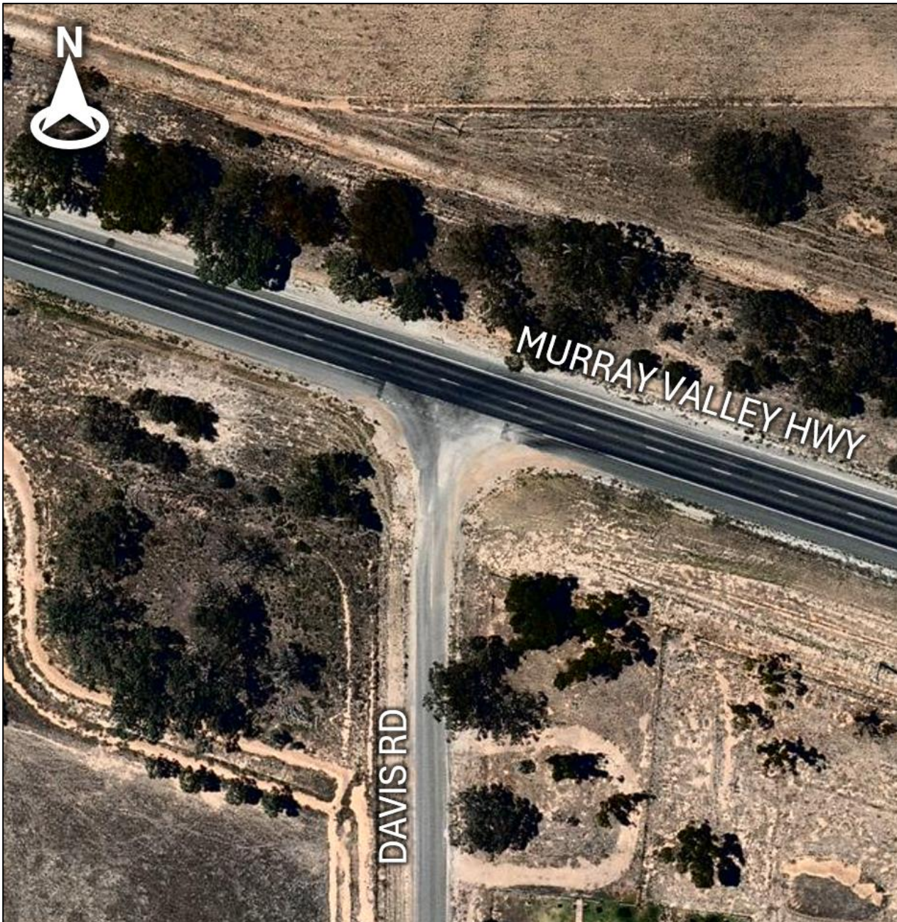
Figure 4-11: Murray Valley Highway / Davis Road intersection
