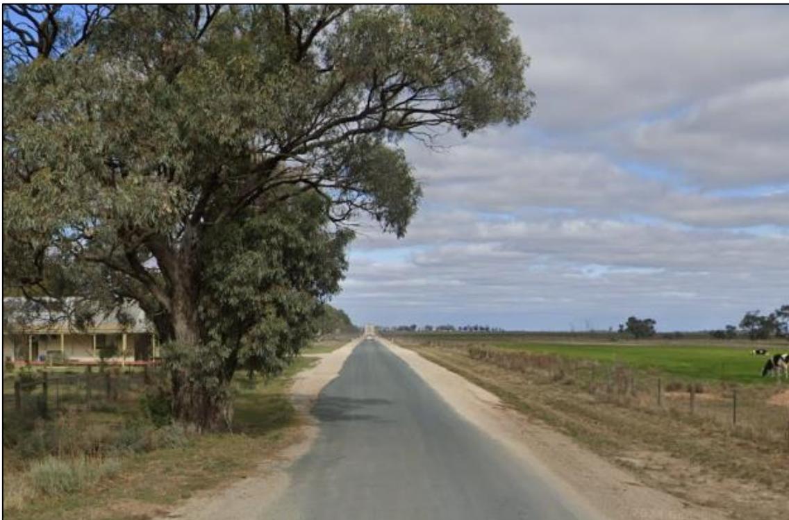
Figure 4-5: Davis Road (looking south from the Murray Valley Highway)
