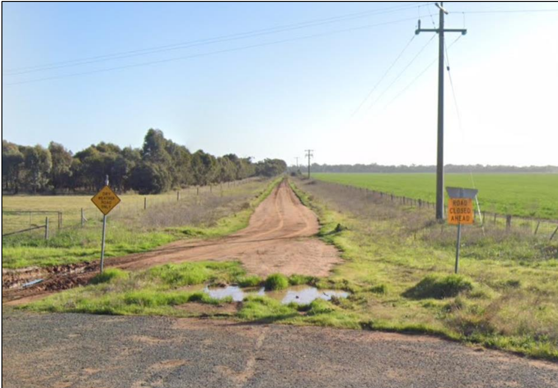
Figure 4-4: Heppell Road (facing north from the Murray Valley Highway)
