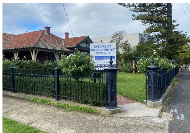
Figure 4-15. Wrought iron fence running adjacent to footpath along property boundary, facing southwest
