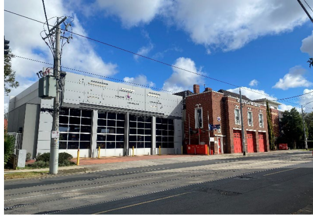
Figure 4-11. Footscray Fire Station Complex, facing west
