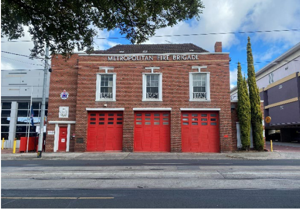
Figure 4-10. Red brick Footscray Fire Station Complex building, facing southwest
