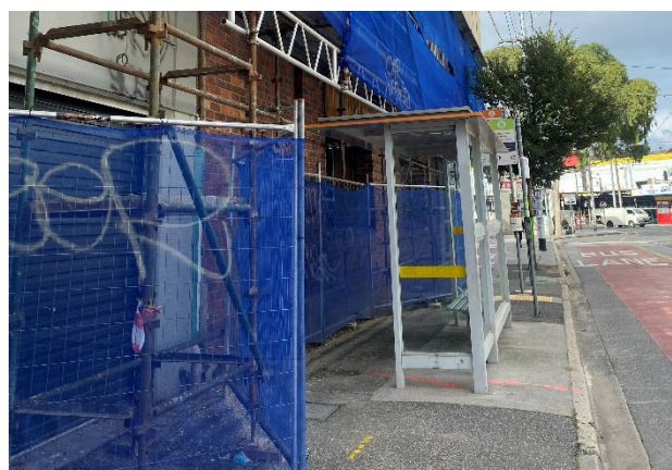
Figure 3-21. 76 Nicholson Street towards tram stop, facing northwest
