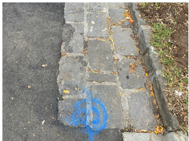
Figure 3-14. Closeup of bluestone kerb and drain at 105 Droop Street (The Crescent), facing southwest
