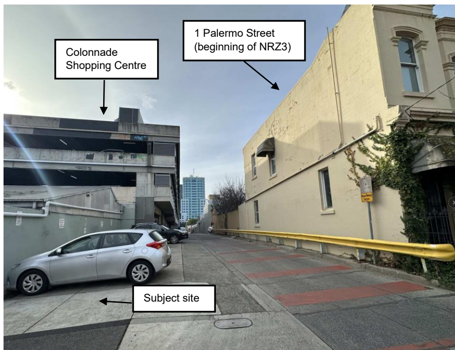
Figure 7: Rear of subject site showing Forster Street and 1 Palermo Street (dwelling)
