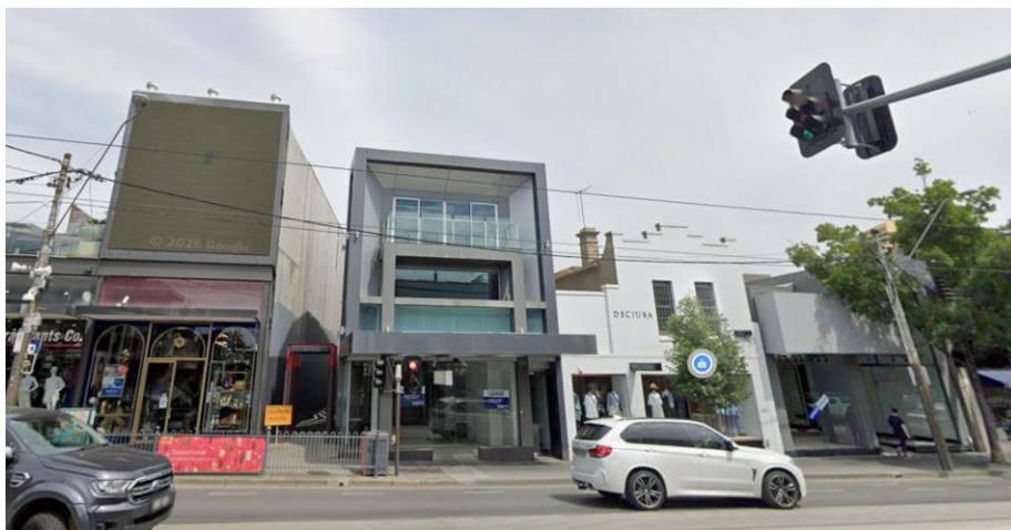
Figure 10: Typical character and form of commercial uses on Chapel Street
