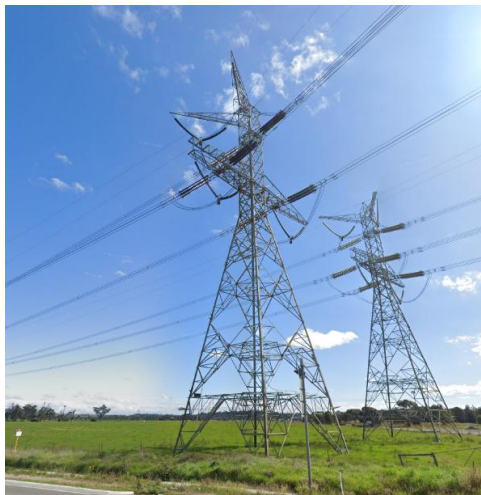
Figure 9 – Typical 500kV pylon.
