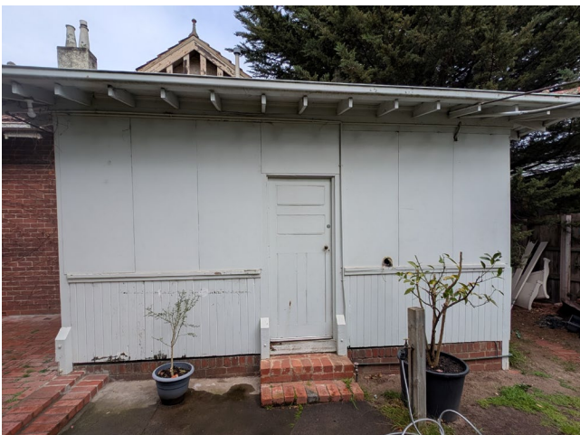
Figure 6 – The northwest (rear) wing.
