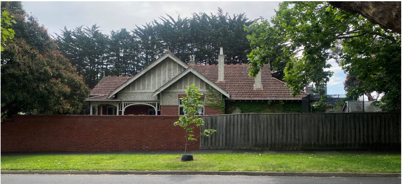
Figure 2 – View of the side façade of the subject building from the opposite side of Scott Street.
