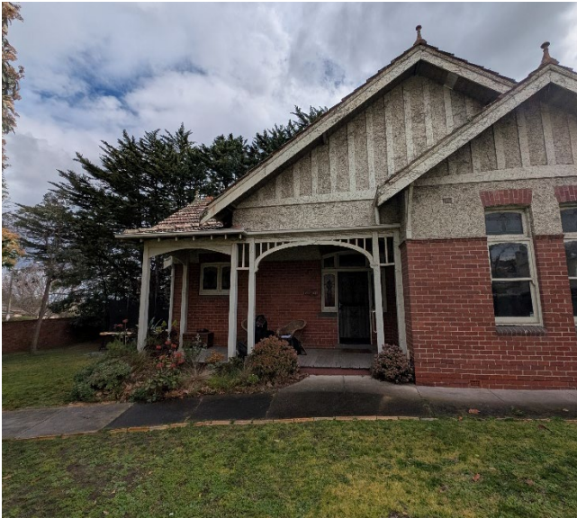
Figure 4 – The southeast (front) corner of the dwelling.
