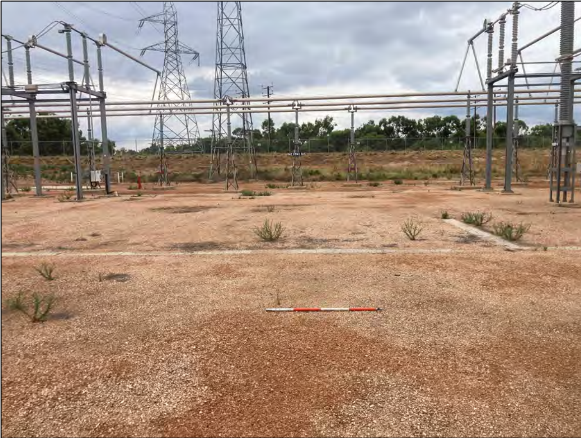
Photo 7: Approximate location of new 220kV Bay. North west orientation. Photo: D.Wall, 2023.
