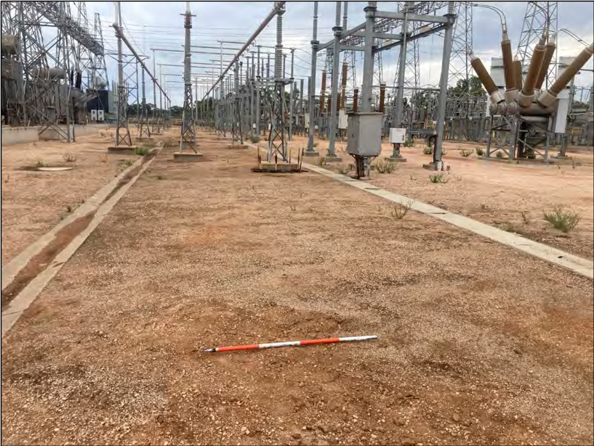
Photo 9: Cleared ground over majority of the site underneath existing power plant. Photo: D.Wall, 2023.
