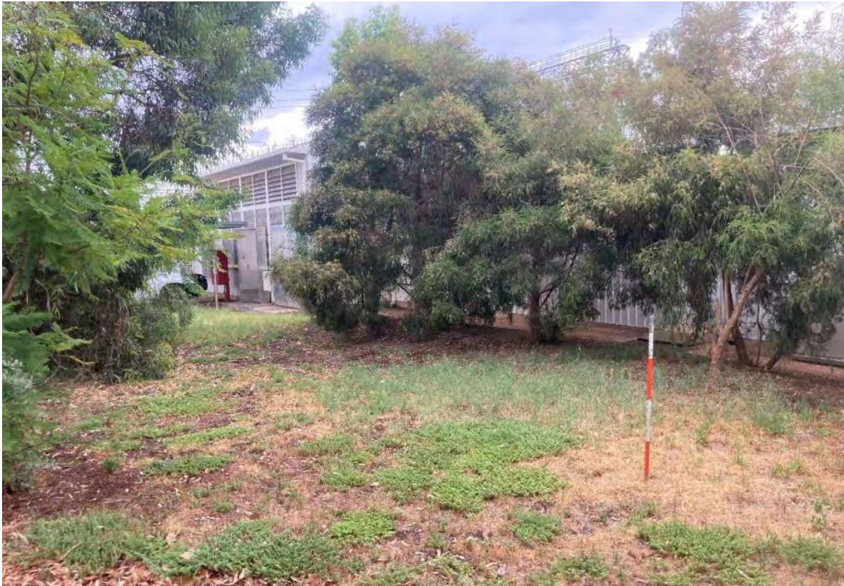
Figure 2 Location of new outdoor battery enclosures, adjacent to existing buildings. North orientation. (Source: Red-Gum Environmental Consulting Aboriginal Cultural Heritage Due Diligence Assessment)
