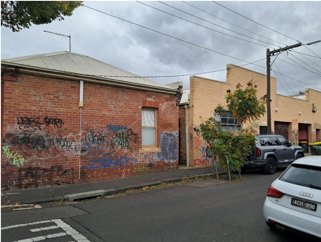
Figure 12: Frontage of heritage building to Argyle Street
