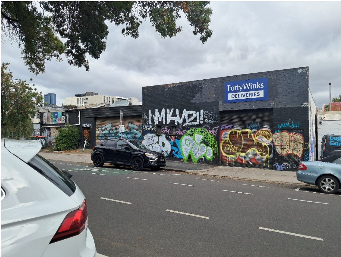
Figure 11: Site frontage to Napier Street
