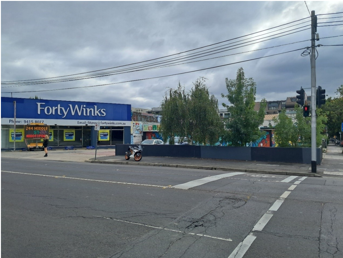
Figure 10: Site frontage to Johnston Street
