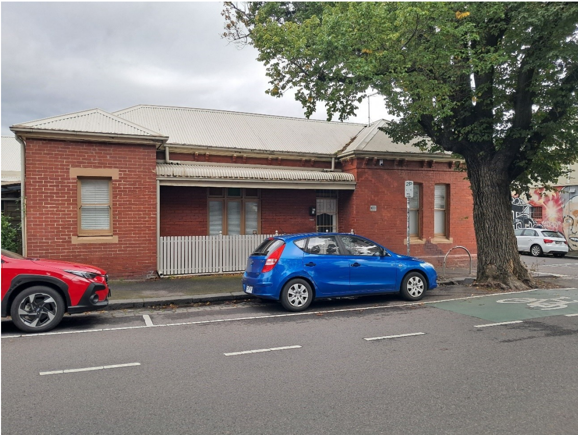
Figure 20: 329 Napier Street frontage to Napier Street (14 April 2026)
