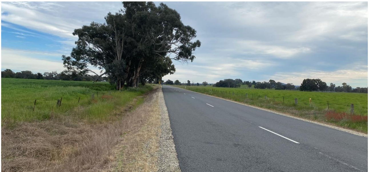
Figure 7 Barnawartha-Howlong Road (facing south)
