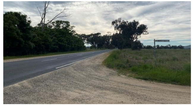
Figure 5 Murray Valley Highway (facing east)
