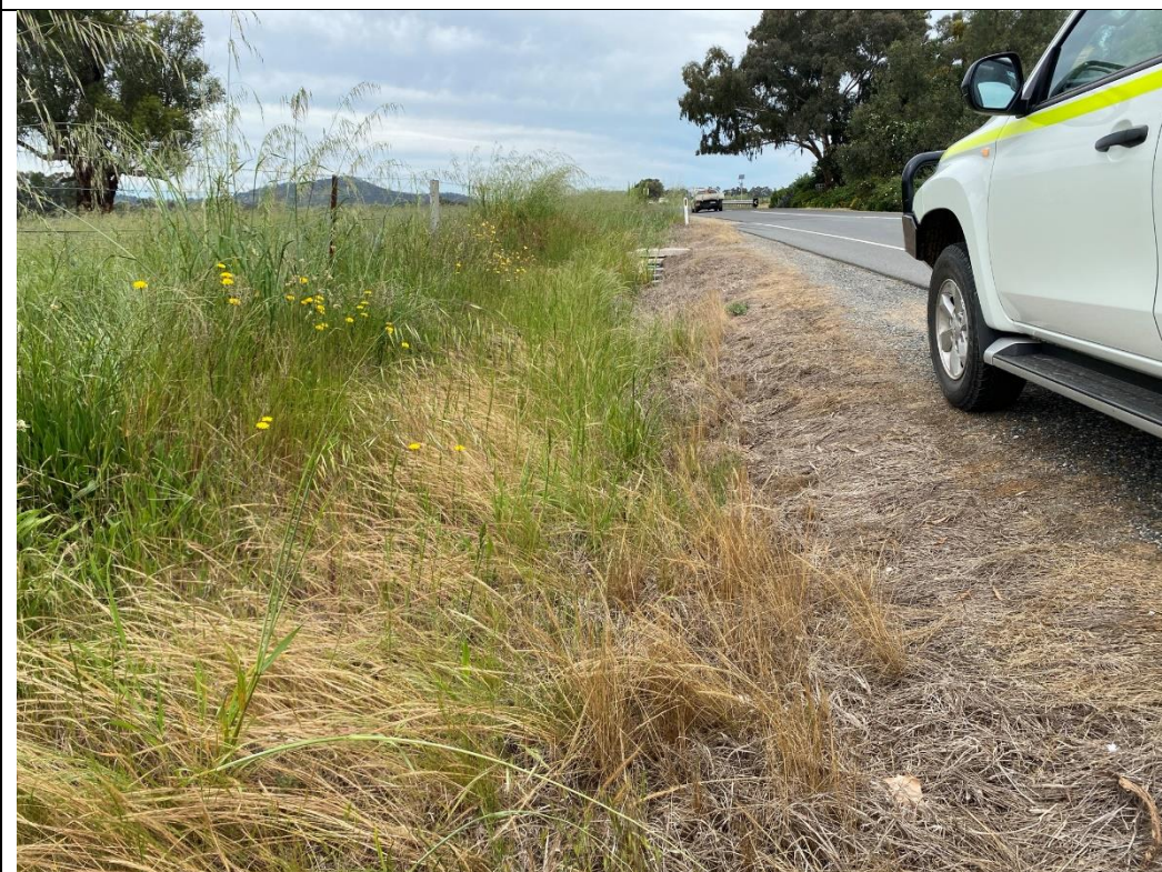
Grassed Swale along Barnawartha Road facing south (corner of Murray Valley Hwy)
