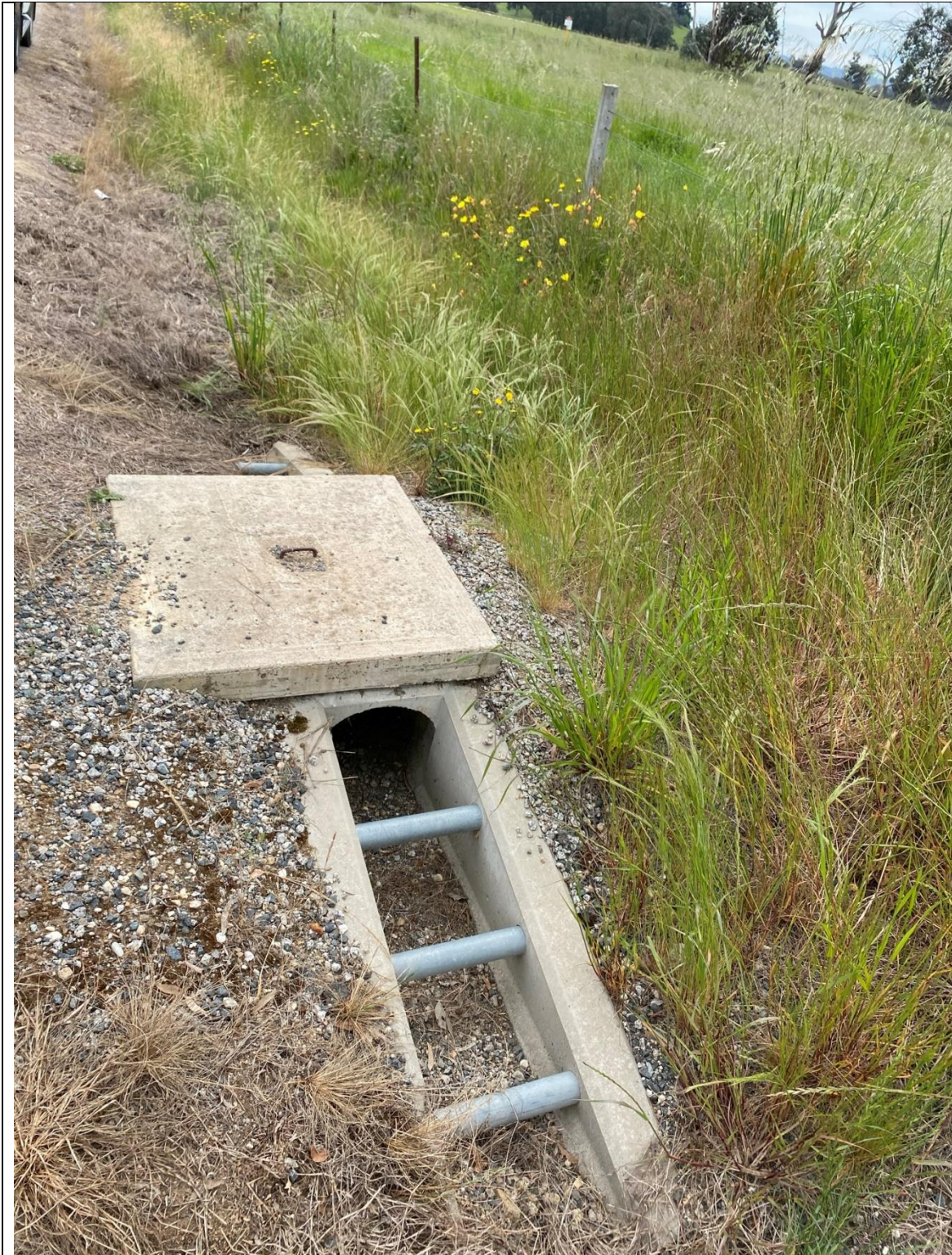
Culvert along Barnawartha Road facing north (corner of Murray Valley Hwy)
