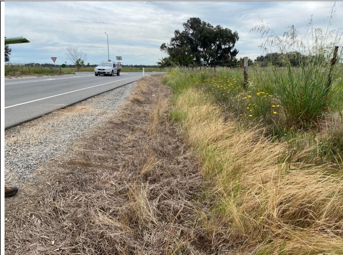
Grassed Swale along Barnawartha Road facing north (corner of Murray Valley Hwy)
