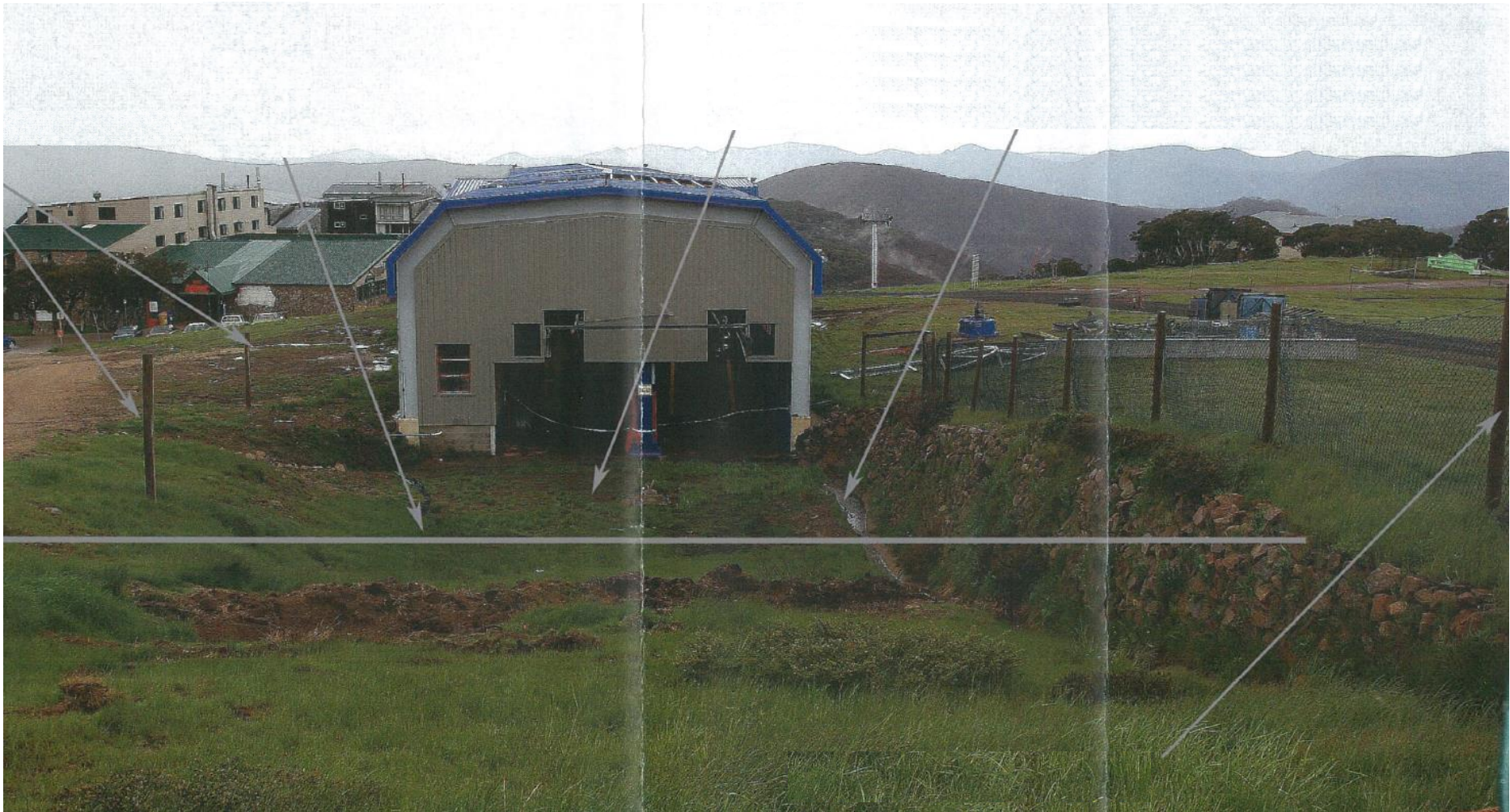
Photo 3 – Western end of Mid-station in 2007 during the removal of the Blue Bullet 2 lift. This western wall end was subsequently boarded up and the excavation backfilled to the levels seen in Photos 1 & 2.
