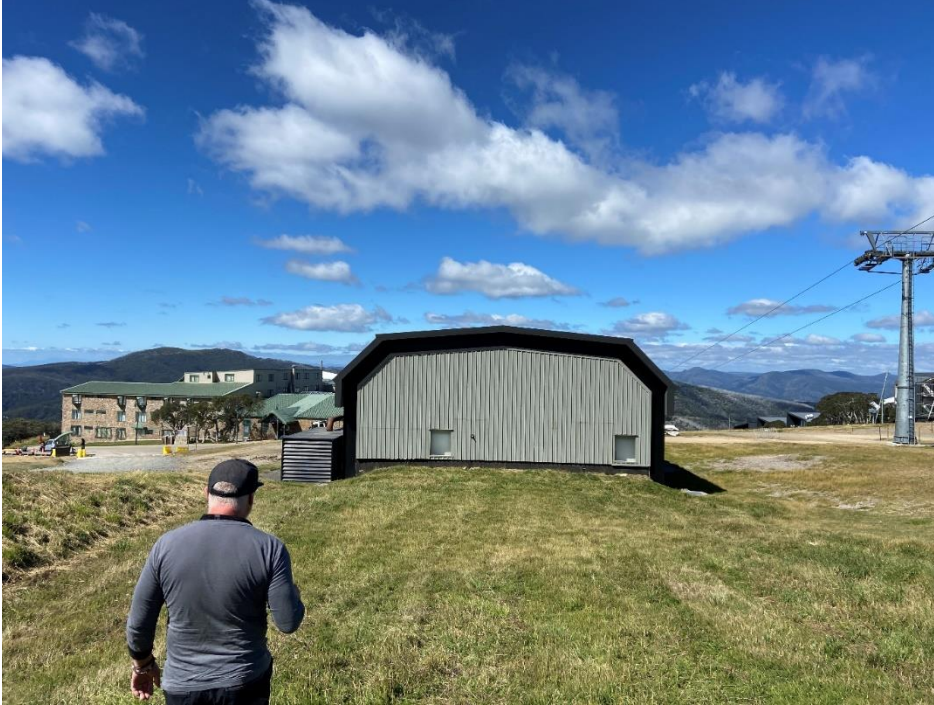
Photo 1 – Western wall of Existing Mid-station building.
