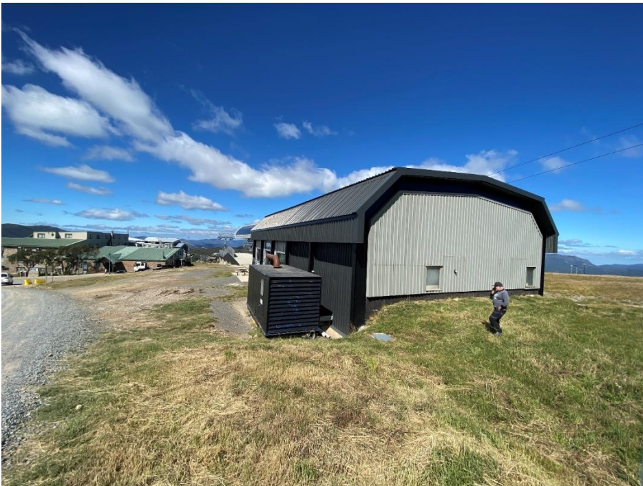
Photo 2 – Western and northern walls of existing Mid-station building.
