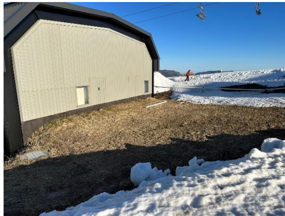
West elevation and vegetation
