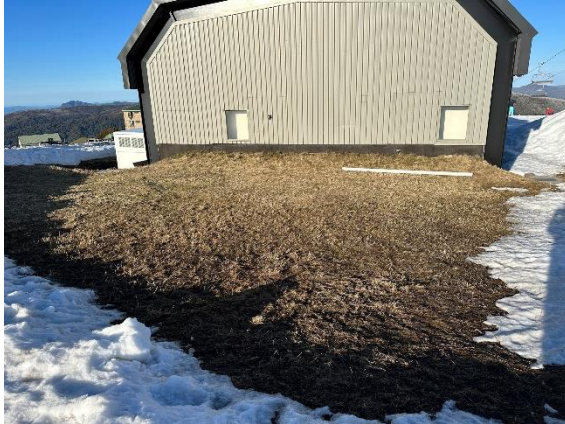
West elevation and vegetation
