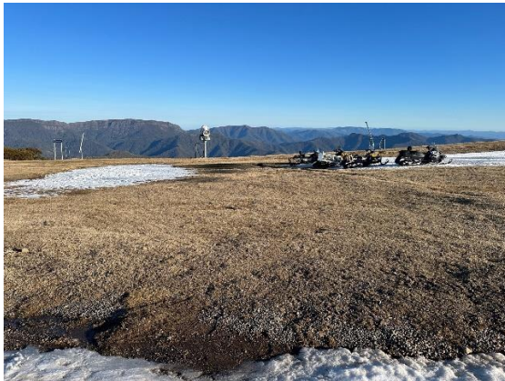
Looking south, southern trenching alignment
