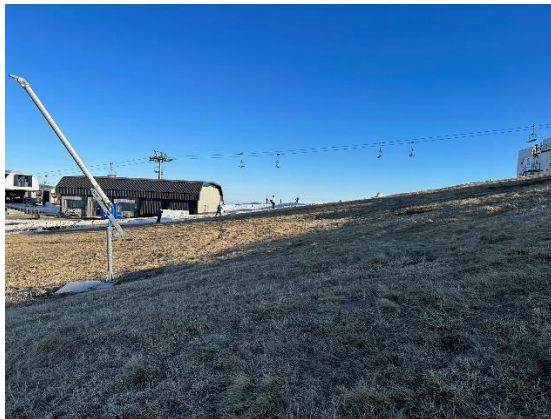
Looking south, northern trenching alignment
