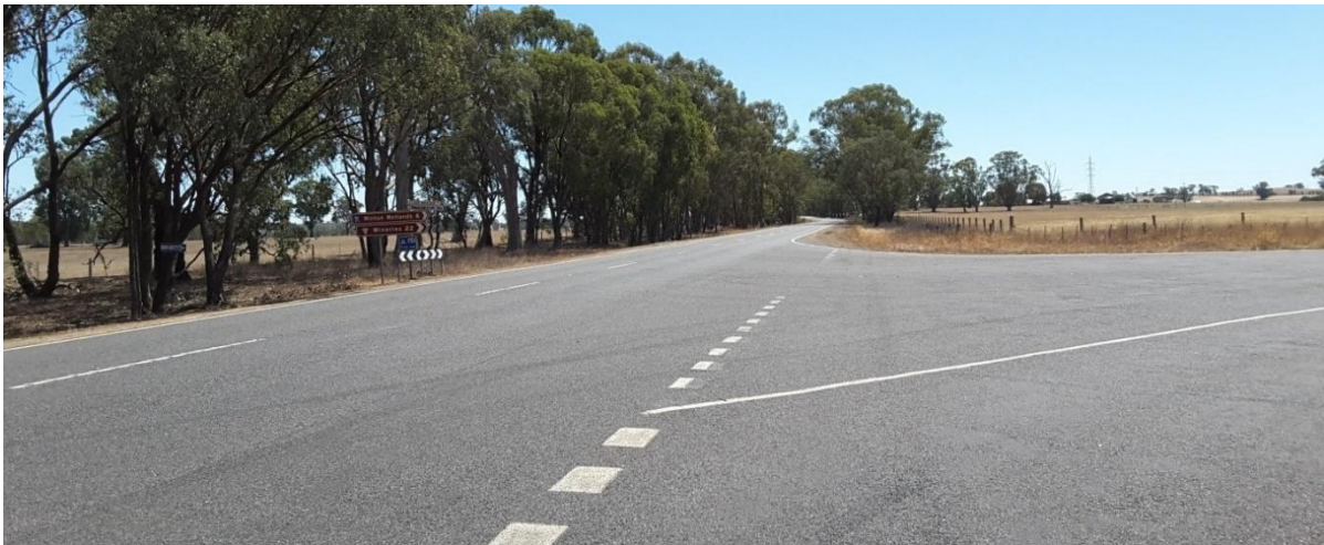
Figure 7 Intersection of Lake Mokoan Road and Benalla-Yarrowonga Road looking northbound
