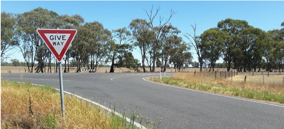
Figure 6 Lake Mokoan Road looking westbound at its crossroad priority intersection with Benalla-Yarrowonga Road
