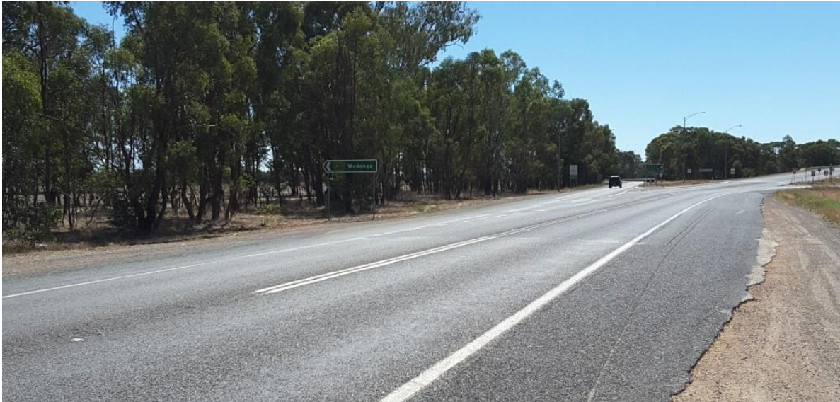
Figure 2 Sydney Road looking towards the Hume Highway interchange
