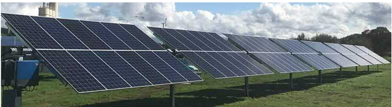
Figure 3 Typical Single Axis Tracking System with Two Modules in Portrait Orientation (Source: SRPS)
