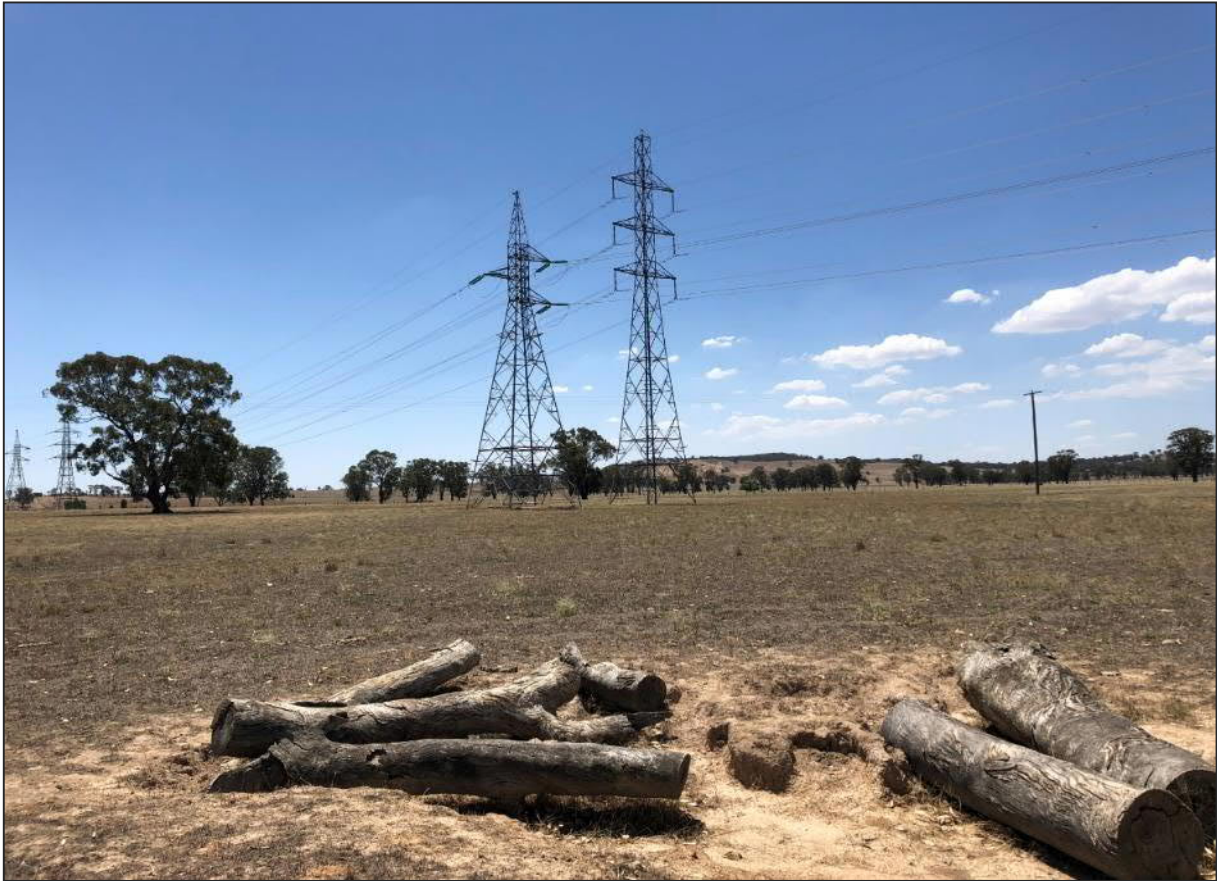
Figure 6: 220 kV Glenrowan to Shepparton transmission line and smaller local feeder line
