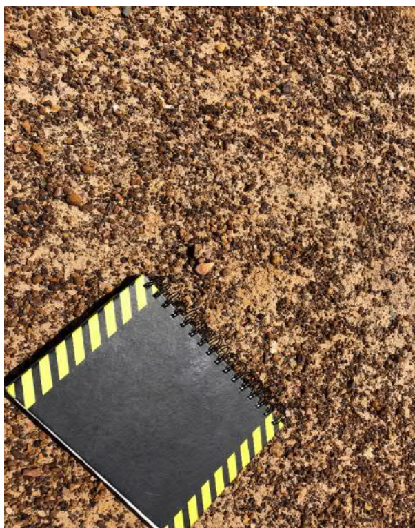
Figure 8: Gravel exposed on farm dam embankment
