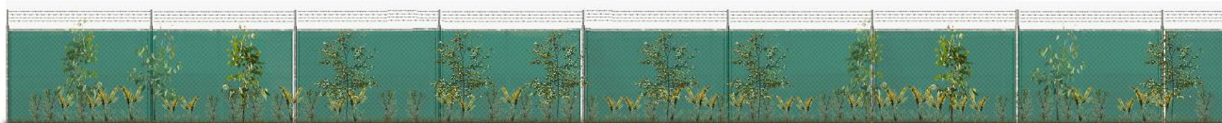
Figure 6 Typical 10m wide screening section - 2 years post installation showing security fence with indicative shade cloth behind
